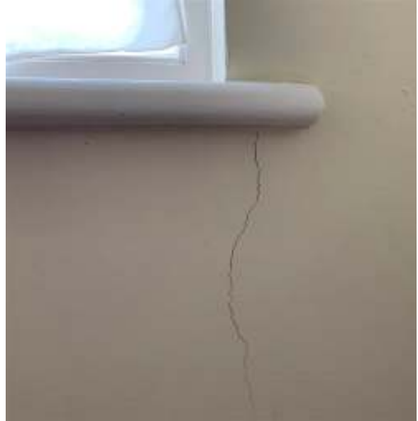
Half-landing - below window on rear wall
