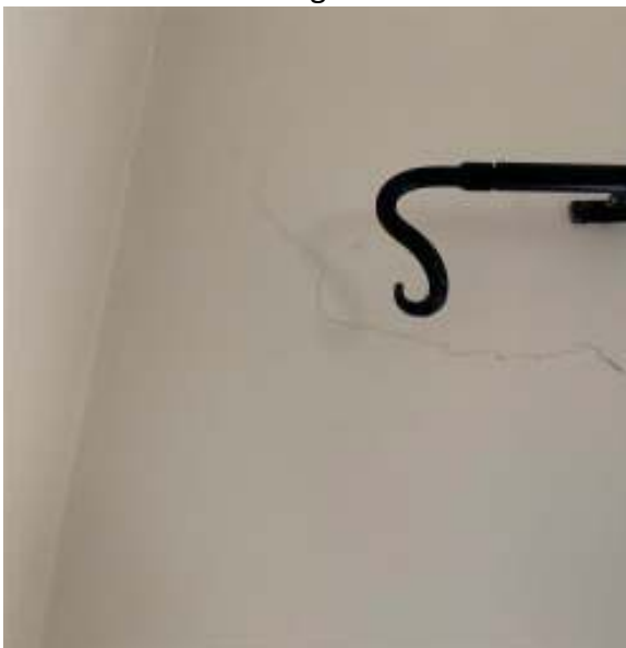
Half landing - above window on rear wall
