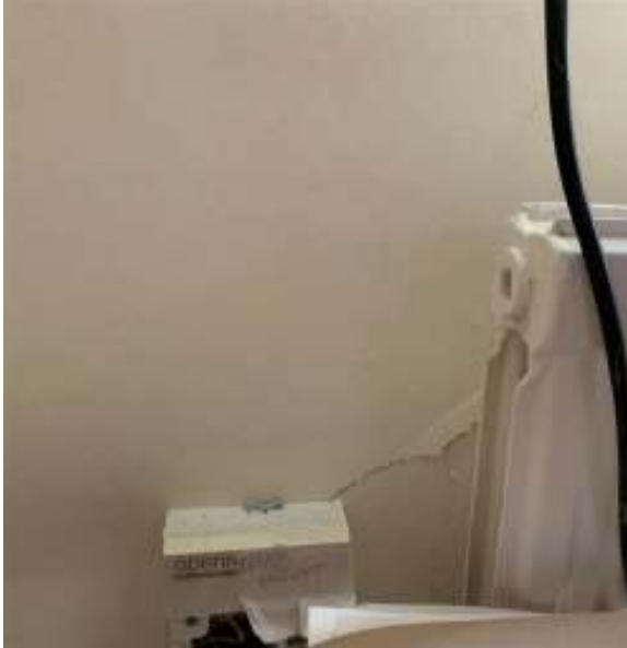
Left reception - below right of window
