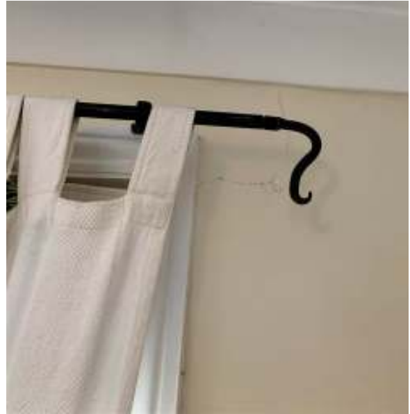
Right reception - above left side of window
