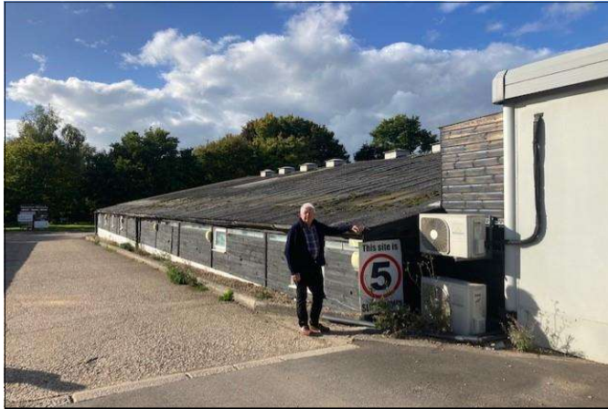
Existing Buildings at Barns Court have very low minimum eaves
