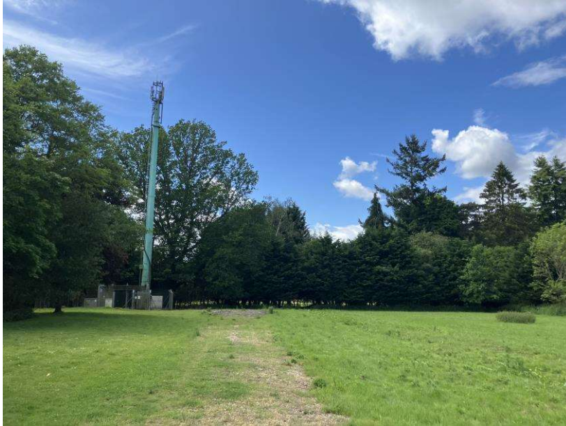
Photo of Phase 1b site, looking west.
