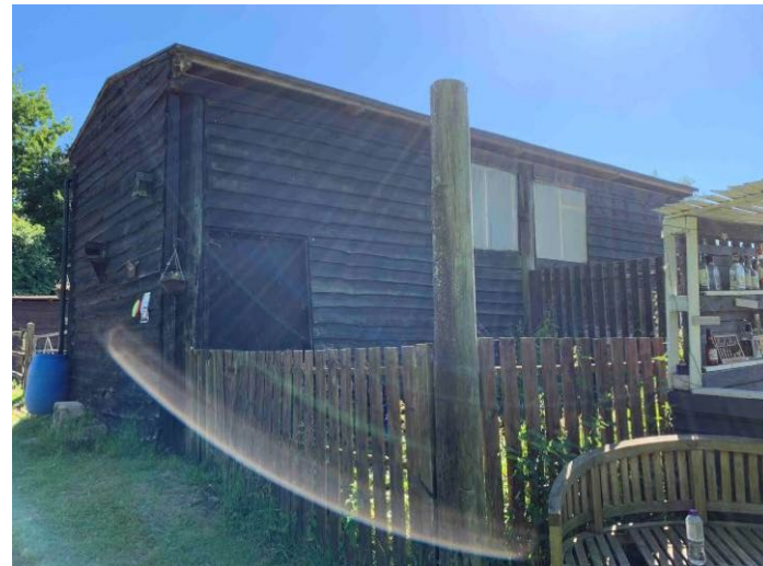
Existing barn – east and north elevations, along with established enclosed area
