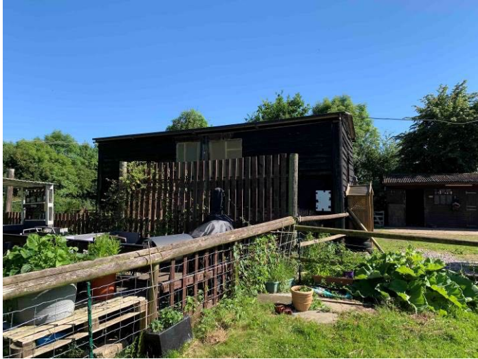
Existing barn - north elevation
