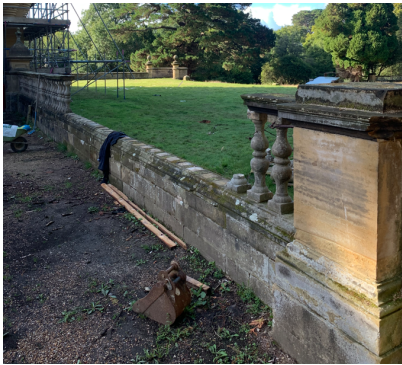
Existing condition of wall
