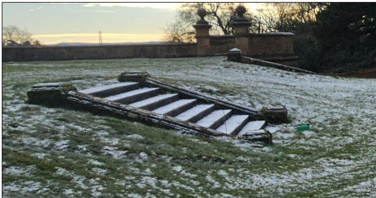
863 Reference Image of Existing steps on site 02 Wykehurst Place
