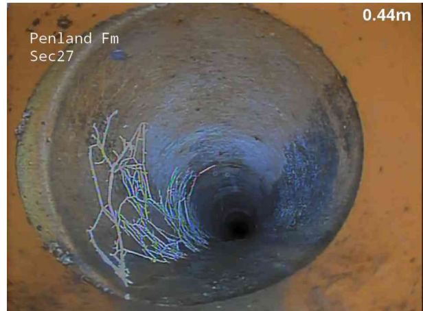
2, 00:00:08, 0.50 m Pipe material changes to vitrified clay at this point
