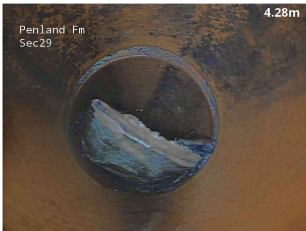
5, 00:00:28, 4.50 m Settled deposits, coarse, 45% cross-sectional area loss
