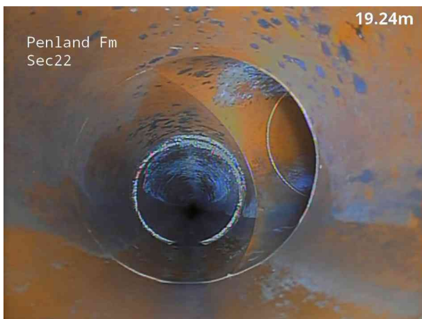
3, 00:00:42, 19.40 m Junction at 3 o'clock, 100mm dia
