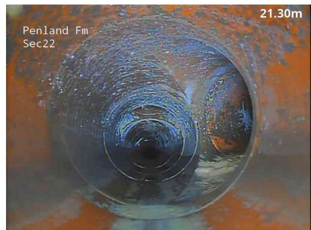
4, 00:00:51, 21.40 m Junction at 3 o'clock, 100mm dia
