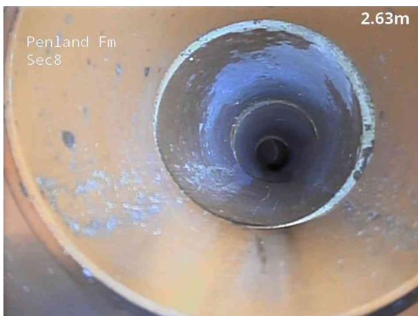
3, 00:00:25, 2.70 m Pipe material changes to vitrified clay at this point
