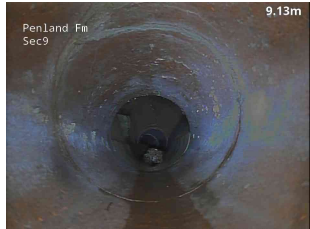
2, 00:01:04, 9.10 m Fracture, circumferential from 12 o'clock to 12 o'clock
