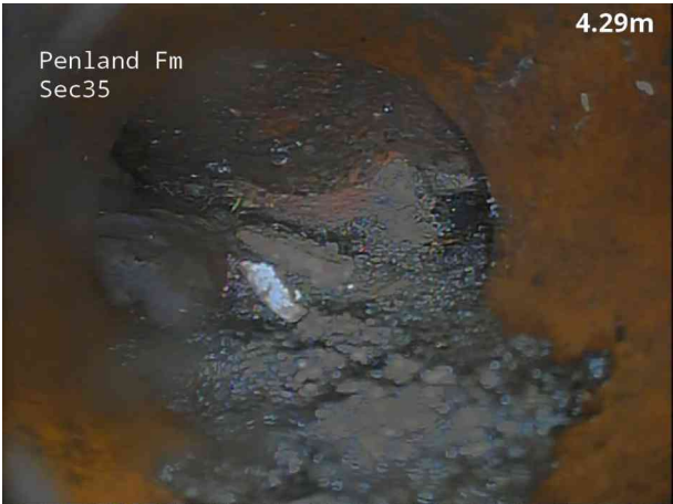
3, 00:00:48, 4.50 m Finish node, soakaway, reference: SK, Assumed Soakaway
