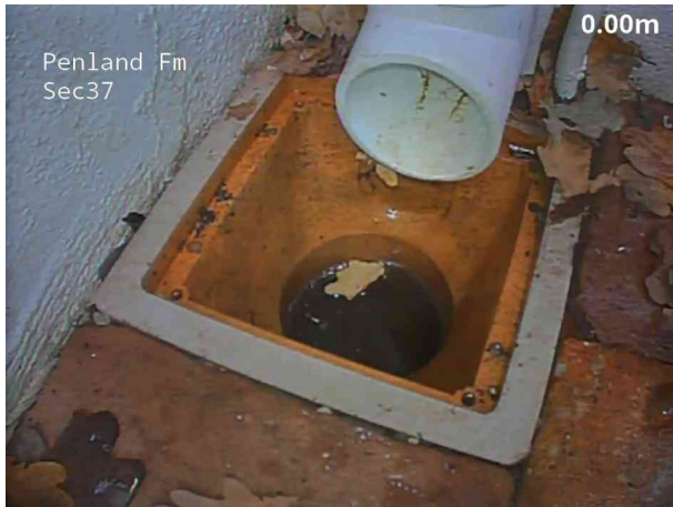
1, 00:00:03, 0.00 m Survey abandoned, Trapped gully, unable to survey
