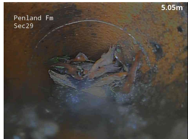
6, 00:00:35, 5.10 m Survey abandoned, Camera compacting debris, possibly serving Surface Water network
