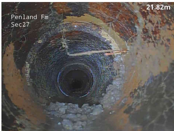
11, 00:02:11, 22.00 m Roots, fine at joint
