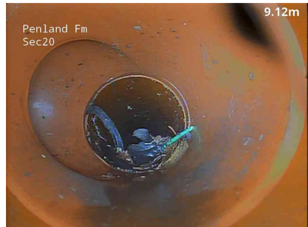
2, 00:00:29, 9.30 m Junction at 9 o'clock, 100mm dia
