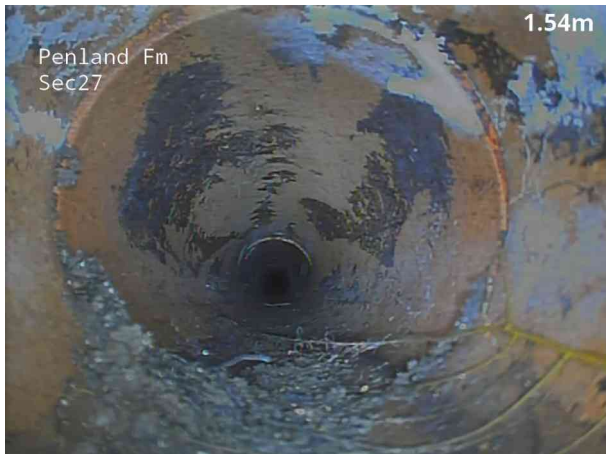
3, 00:00:15, 1.60 m Roots, fine at joint
