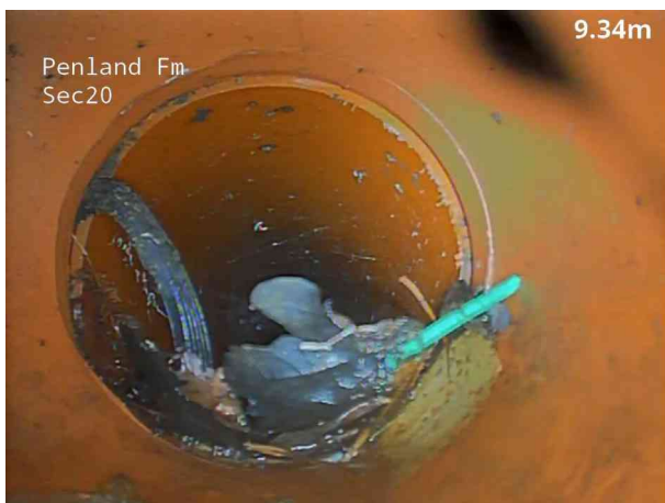
3, 00:00:32, 9.40 m Sealing ring intruding, loop hanging below centre from 7 o'clock to 10 o'clock
