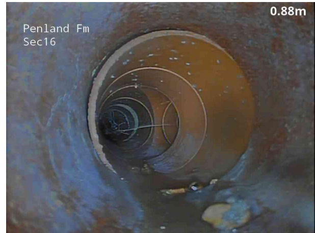
2, 00:00:14, 1.00 m Pipe material changes to polyvinyl chloride at this point
