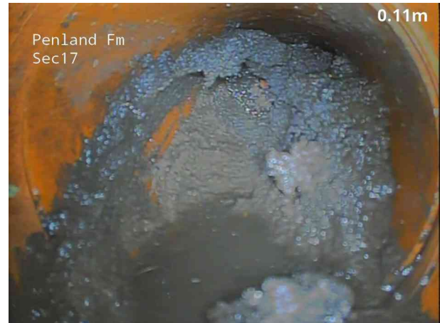
2, 00:00:13, 0.20 m Settled deposits, fine, 90% cross-sectional area loss
