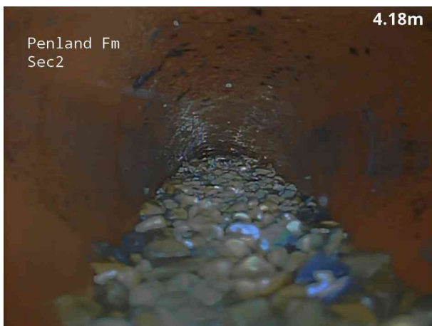
3, 00:00:21, 4.20 m Settled deposits, coarse, 10% cross-sectional area loss, start
