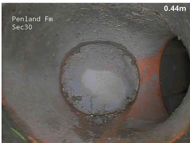
3, 00:00:24, 0.60 m Junction at 3 o'clock, 100mm dia
