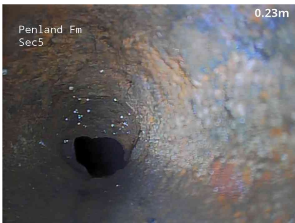
3, 00:00:07, 0.40 m Pipe material changes to cast iron at this point
