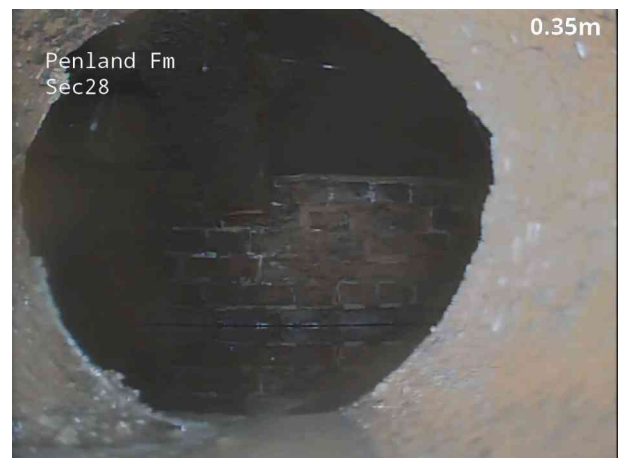
4, 00:00:11, 0.50 m General remark, Dipper pipe missing
