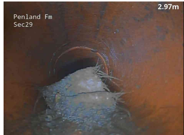
4, 00:00:21, 3.00 m Roots, mass, 10% cross-sectional area loss
