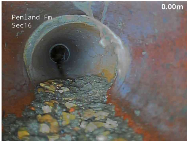
1, 00:00:04, 0.00 m Settled deposits, coarse, 10% cross-sectional area loss
