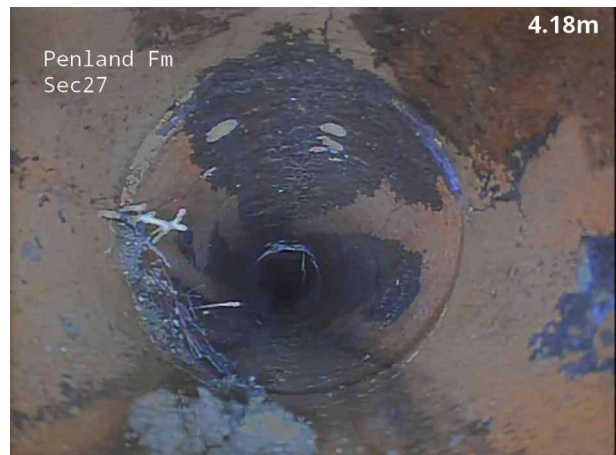
6, 00:00:33, 4.30 m Roots, fine at joint, start
