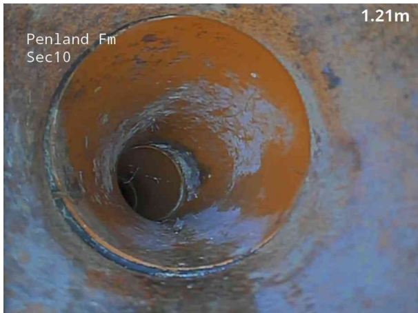
3, 00:00:25, 1.30 m Pipe material changes to polyvinyl chloride at this point
