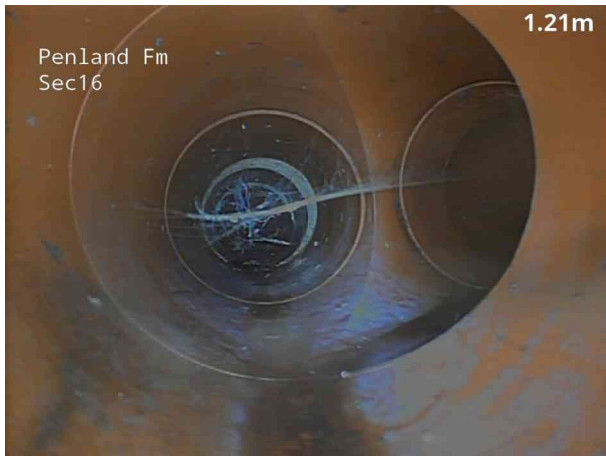
3, 00:00:18, 1.30 m Junction at 3 o'clock, 100mm dia
