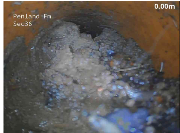
2, 00:00:34, 0.10 m Settled deposits, fine, 95% cross-sectional area loss
