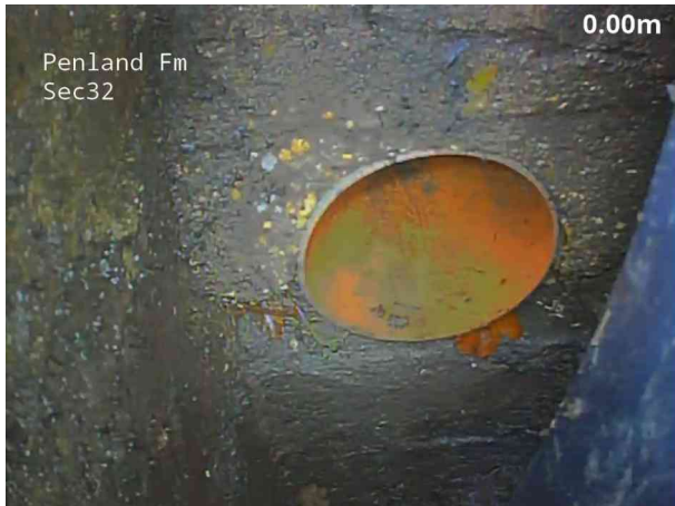
1, 00:00:00, 0.00 m Start node, outfall, reference: OF1, Retro fitted relief pipe
