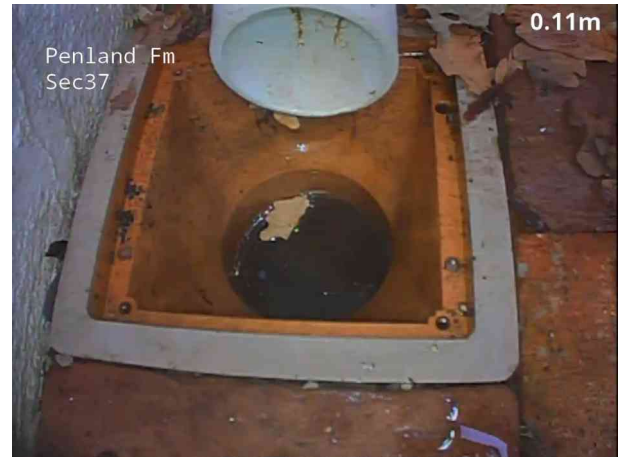
2, 00:00:03, 0.00 m Survey abandoned, Trapped gully, unable to survey
