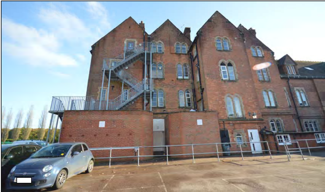
Plate 11: The northwest side of the North School showing the further gable to the group added in 1937 (behind the fire escape)
