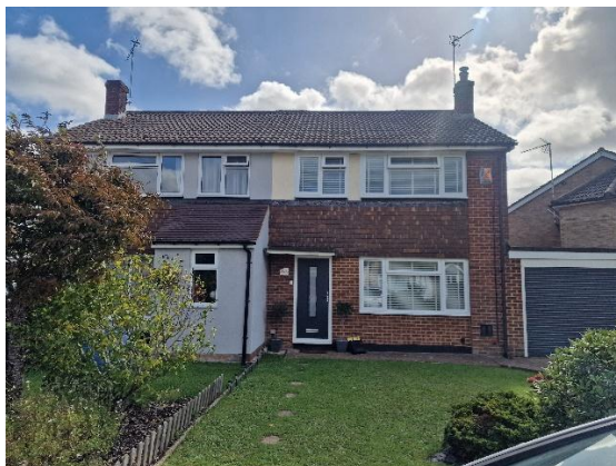
Principal (north west) elevation
