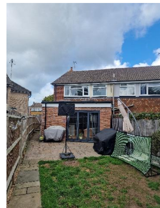
Rear (south east) elevation
