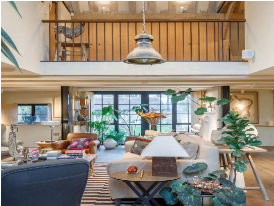
Light touch metal spindles with timber handrail
