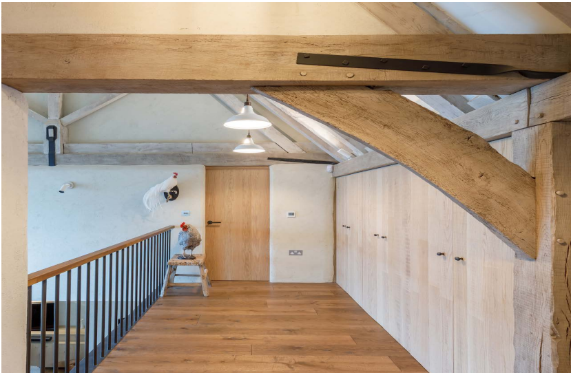
Light touch metal spindles with timber handrail
