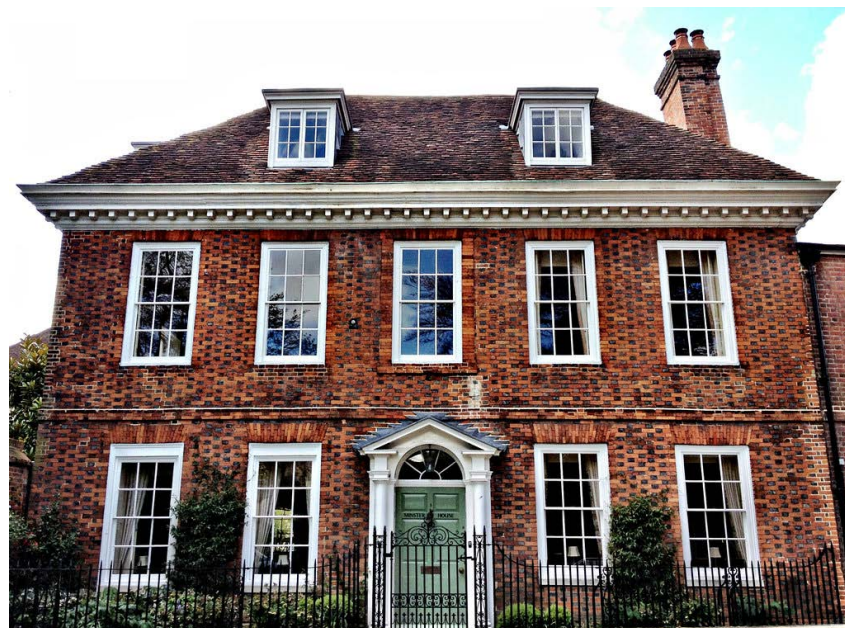
Georgian Home with Flat Lead Roof Dormers
