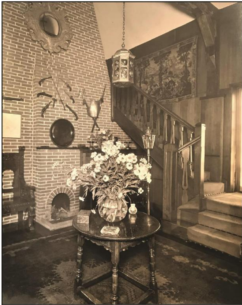
Images from the latest heritage statement showcase the 1920s addition stair balustrade and spindles and in place.
