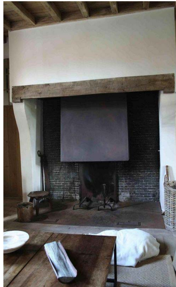
Chimney canopy to existing fireplace.
