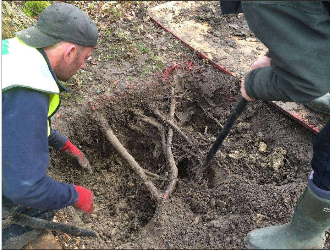
Fig. 3 Initial manual dig exercise and root exposure and treatment as necessary
