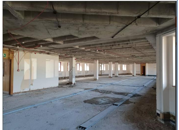
Photo 19: Internal View of the Building
