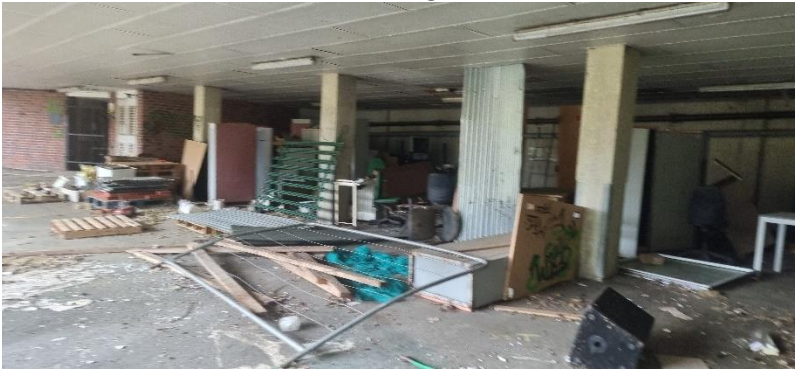
Photo 7: Undercover Car Park Area to the Northwest of the Building.
