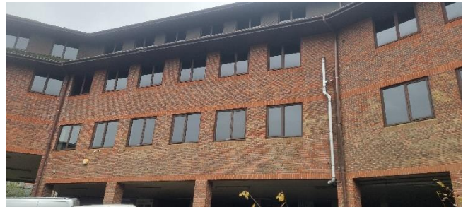
Photo 15: Northwestern Elevation of Site.
