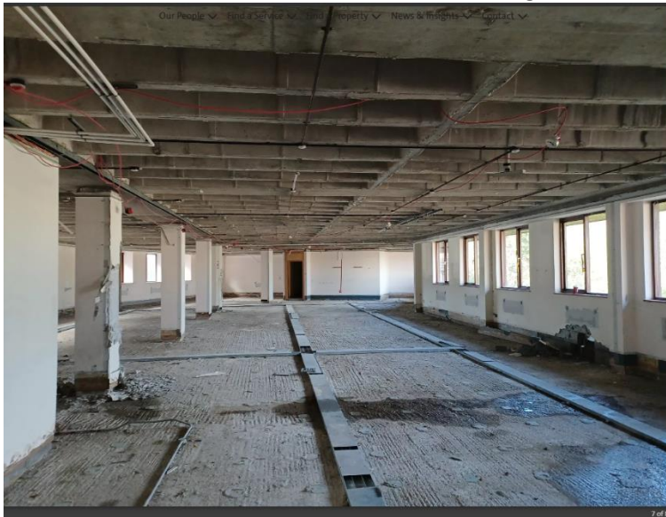
Photo 18: Internal View of the Building
