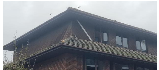
Photo 9: Southwestern Corner of the Building.
