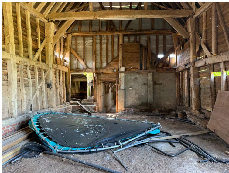
Image 9: Internal view of Building B2.
