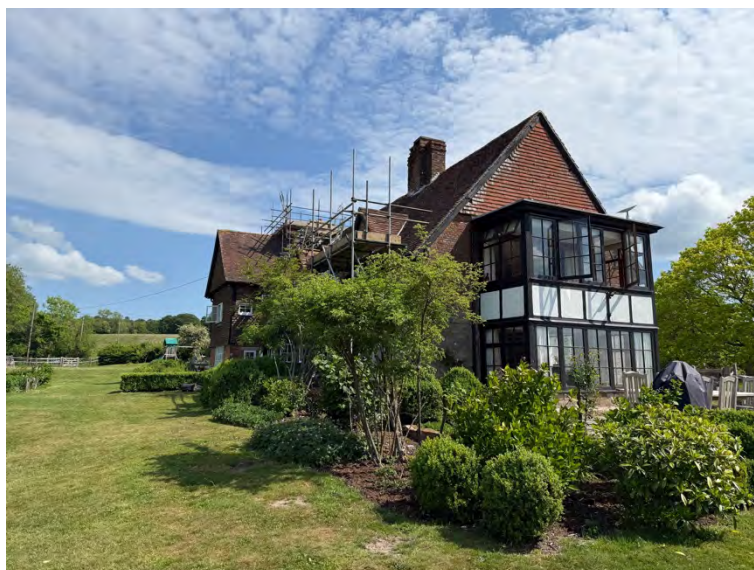
Image 8: Hanging tiles on the southern elevation of B1.
