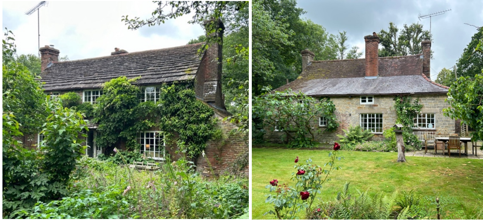
The front range with its Horsham slate roof and the rear range in slate.
