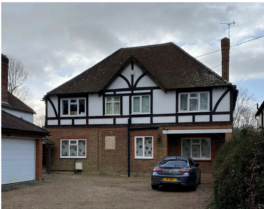
Figure 6 – Existing dwelling at 64 Folders Lane
