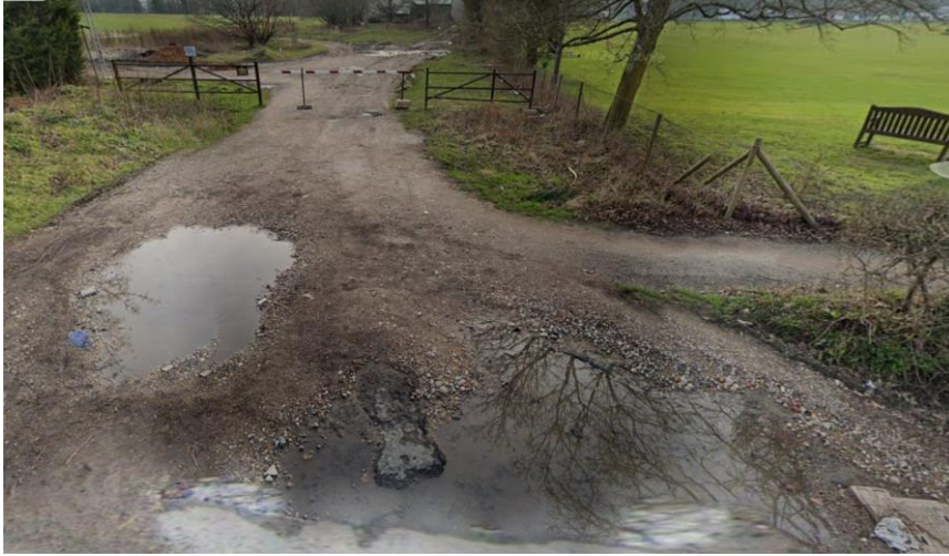
Figure 3.5 Site Access looking west from access
