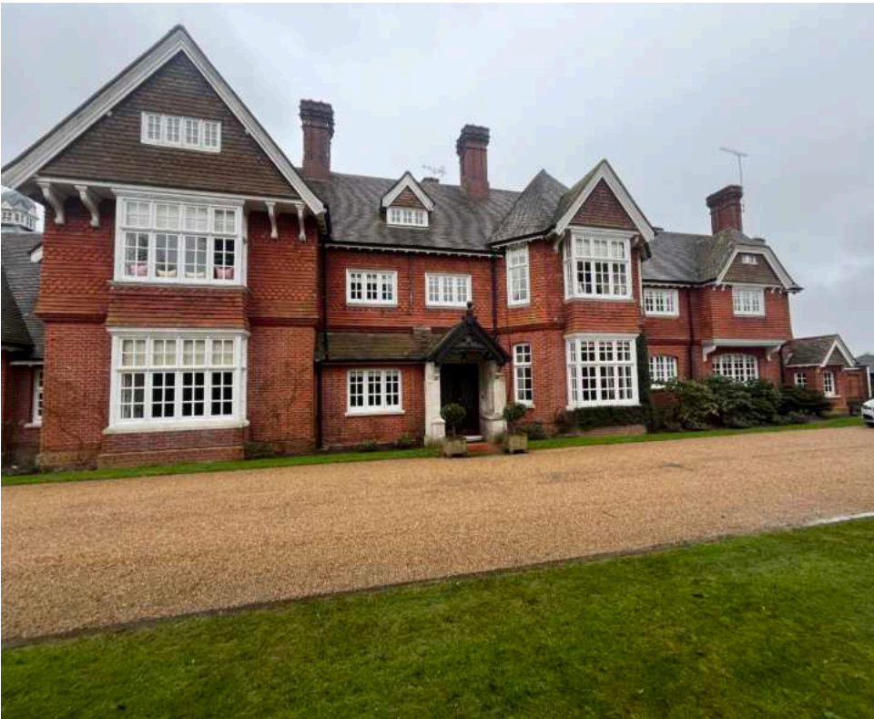
West elevation of the house
