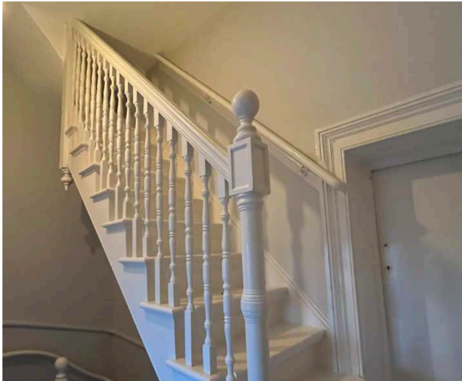
Staircase leading to now demolished tower and blocked opening.
