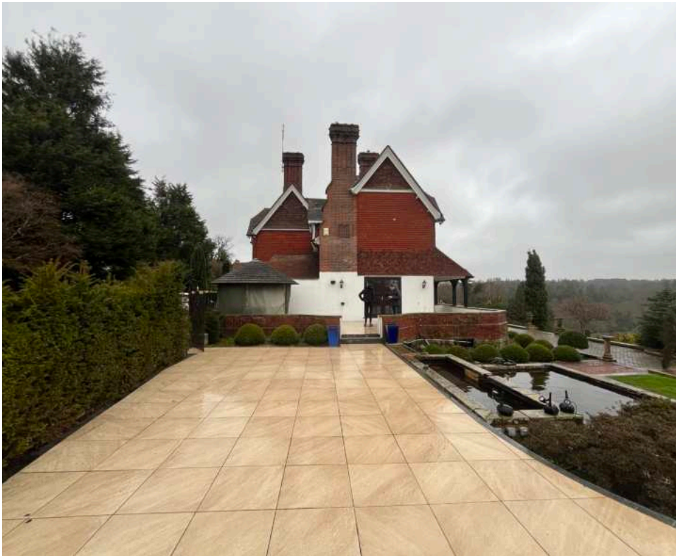
South elevation of the house, patio terrace and dwarf wall
