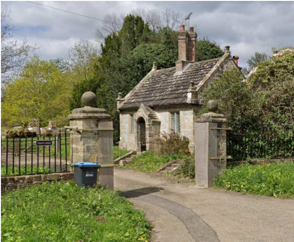
Grade II Listed Gateway at South Lodge
