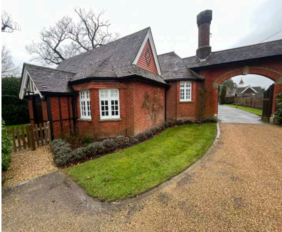
North lodge looking north and brick archway
