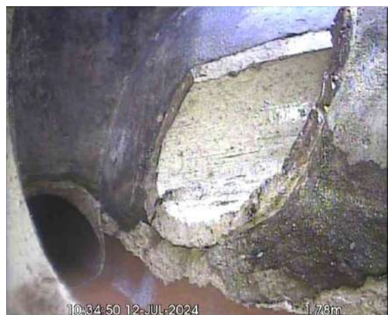
MH1X_d3684f66-d33d-414b-8bac-5e46a45db65e_20240725_091013_389.jpg, 00:00:48, 1.78 m Finish node, manhole, reference: MANHOLE 2 (MH2)
