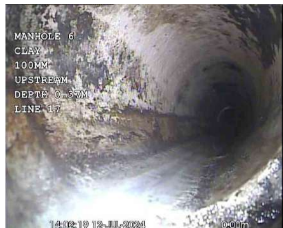
GULLYX_cf37c378-d01c-4b94-8619-aecae9d0c76e_20240725_101301_448.jpg, 00:00:30, 0.00 m Water level, 0% of the vertical dimension
