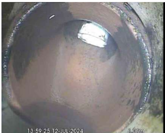
BASINX_40e5934f-6751-4c2f-8103-7d817af70ed0_20240725_101004_289.jpg, 00:00:28, 1.01 m Line deviates up, REST BEND
