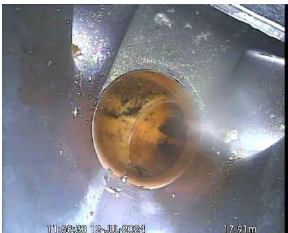
MH2X_acdd8251-032e-4fda-a1d3-9a0cfadee0a2_20240725_093304_170.jpg, 00:02:27, 17.91 m Finish node, manhole, reference: MANHOLE 4 (MH4)
