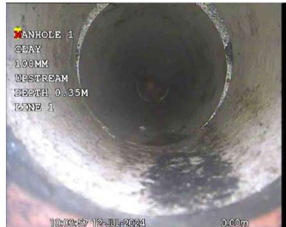
GULLYX_1c9e483a-3e61-4e7c-9347-20a48706a5b3_20240725_090134_214.jpg, 00:00:34, 0.00 m Water level, 0% of the vertical dimension
