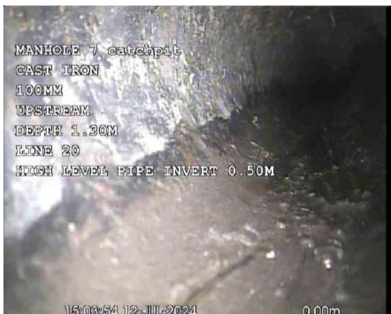
MANHOLEX_092f6c46-9f5c-4244-a0a7-58e180fb86e7_20240725_102110_815.jpg, 00:00:25, 0.00 m Start node, catchpit, reference: MANHOLE 7 (MH7) - CATCHPIT (CP), (HIGH LEVEL PIPE - INVERT - 0.50M)
