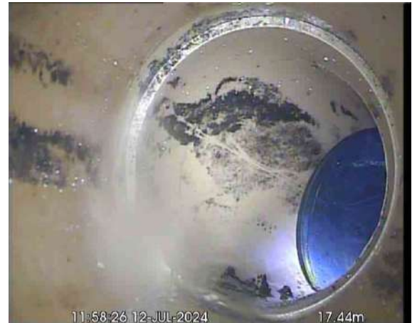
MH2X_ecbc01d4-5401-430c-a4cc-4e8128ef4209_20240725_093238_853.jpg, 00:02:20, 17.44 m Line deviates right
