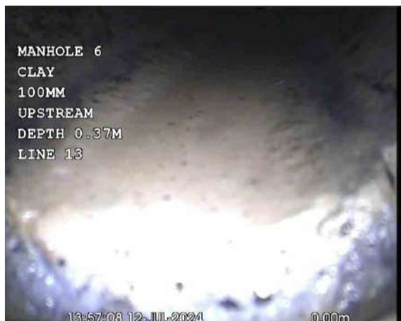
GULLYX_3ca80480-fda7-476d-bdd4-121782959120_20240725_095710_019.jpg, 00:00:22, 0.00 m Start node, manhole, reference: MANHOLE 6 (MH6)
