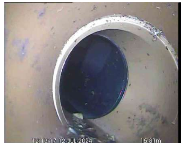
MH4X_9d8f4504-f323-432b-9698-14d451cd618f_20240725_094016_482.jpg, 00:01:29, 15.81 m Line deviates left
