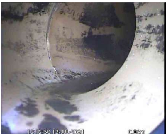
MH4X_047d0d34-fc87-401f-a4c3-3433783703f4_20240725_093918_923.jpg, 00:00:42, 0.06 m Line deviates right
