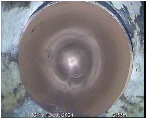
GULLYX_28ba29e2-e34d-48d9-9e89-110dddac1be6_20240725_101336_880.jpg, 00:01:00, 2.53 m Material changes to polyvinyl chloride
