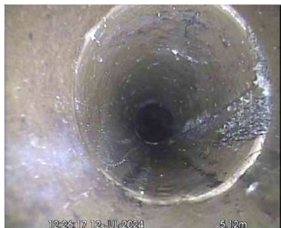
MH5X_109efa46-164d-464f-96dd-18bcad47188e_20240725_094816_811.jpg, 00:01:44, 5.12 m Roots, fine at joint
