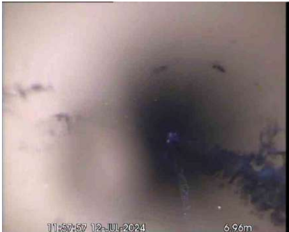
MH2X_88b39d42-4c30-4654-8841-754422e4dc7a_20240725_093224_970.jpg, 00:01:50, 6.96 m Water level, 0% of the vertical dimension
