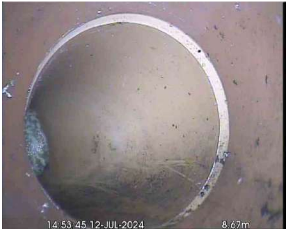
RWDPX_9497cd0e-eee7-4c16-afb8-0b0c38f1904e_20240725_101729_175.jpg, 00:01:16, 8.67 m Line deviates left
