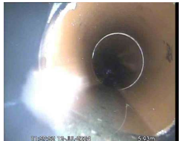
MH2X_2c7dd602-37a2-429a-a2ab-0279f14f5071_20240725_093210_012.jpg, 00:01:46, 5.93 m Water level, 5% of the vertical dimension
