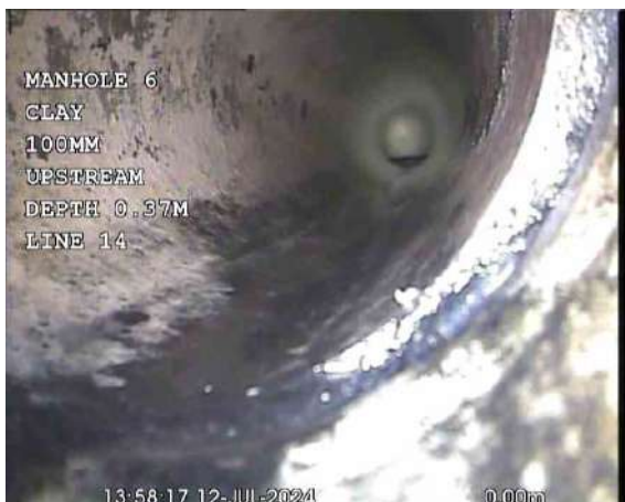
GULLYX_4ba6a257-bb96-4b74-8e54-361352db541e_20240725_095949_671.jpg, 00:00:12, 0.00 m Start node, manhole, reference: MANHOLE 6 (MH6)
