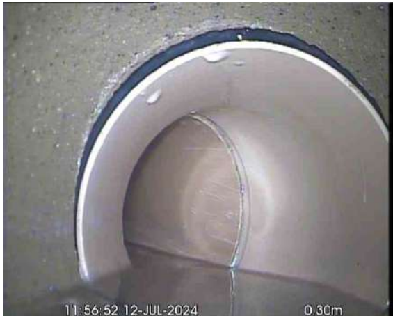
MH2X_b91b3937-c37a-452d-9c54-7c35945f681d_20240725_092617_600.jpg, 00:00:56, 0.30 m Material changes to polyvinyl chloride
