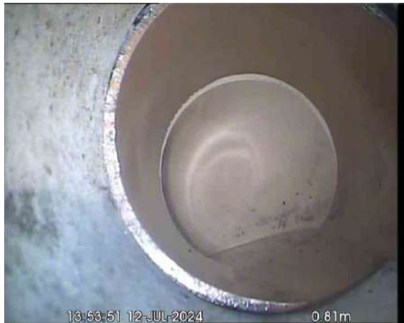
SVPX_6dc84003-04ba-4f4b-a2bc-ade636d85d44_20240725_095258_153.jpg, 00:00:43, 0.81 m Material changes to polyvinyl chloride
