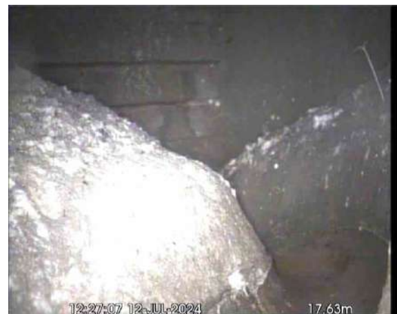
MH5X_14be63c4-1844-4b3b-8d9d-02ec269f888d_20240725_095012_235.jpg, 00:02:35, 17.63 m Finish node, manhole, reference: MANHOLE A (MHA), (DAWN RISE ROAD)
