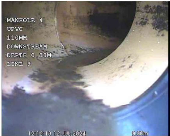
MH4X_55d14c4d-fdbe-480a-a8d1-3ec7317d0af8_20240725_093843_347.jpg, 00:00:26, 0.00 m Start node, manhole, reference: MANHOLE 4 (MH4)
