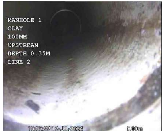
W_CX_471e1211-220d-4303-95f7-17451f9caf6b_20240725_090348_835.jpg, 00:00:20, 0.00 m Water level, 0% of the vertical dimension
