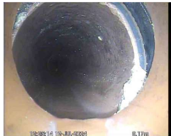
MH5X_f2943572-daea-4cc0-b643-02d9ae5cd5ee_20240725_094641_129.jpg, 00:00:44, 0.17 m Material changes to vitrified clay
