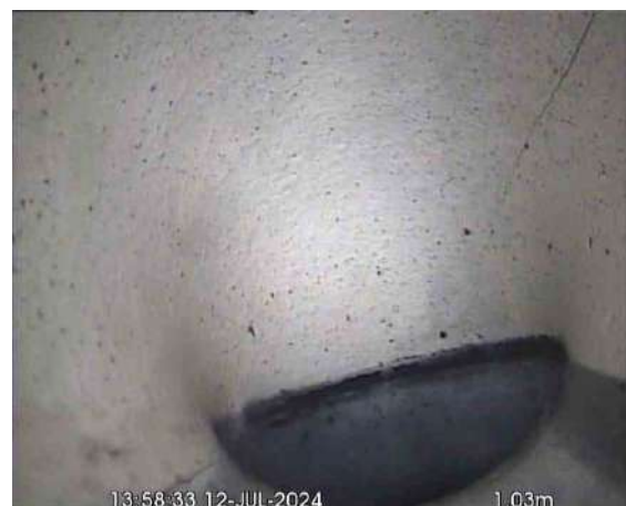
GULLYX_c67647b2-92e2-40c2-a9d7-fb213594d517_20240725_100025_314.jpg, 00:00:28, 1.03 m Finish node, gully, reference: GULLY
