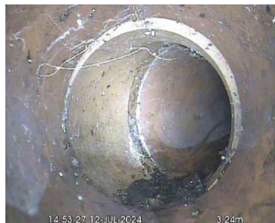
RWDPX_b04b44a7-7c3f-4146-a3f3-0906ec81aae0_20240725_101714_425.jpg, 00:00:58, 3.24 m Line deviates right
