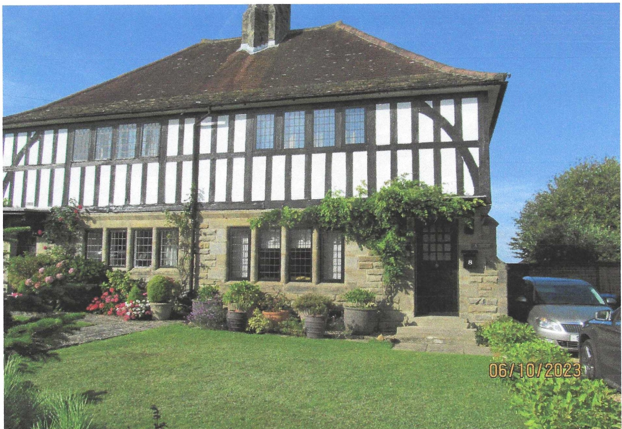
No 8 Newstone Cottages from road frontage
