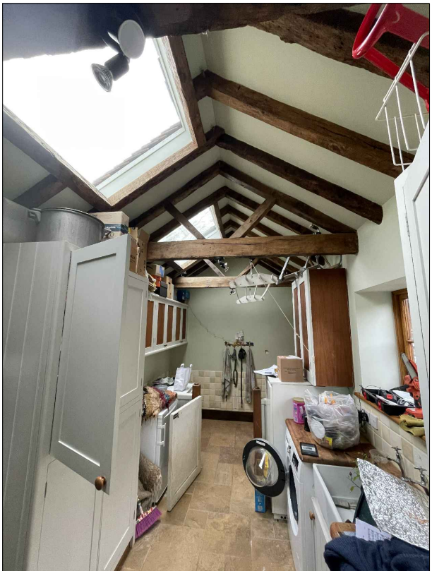
PHOTOS OF EXISTING ROOFLIGHTS IN UTILITY
