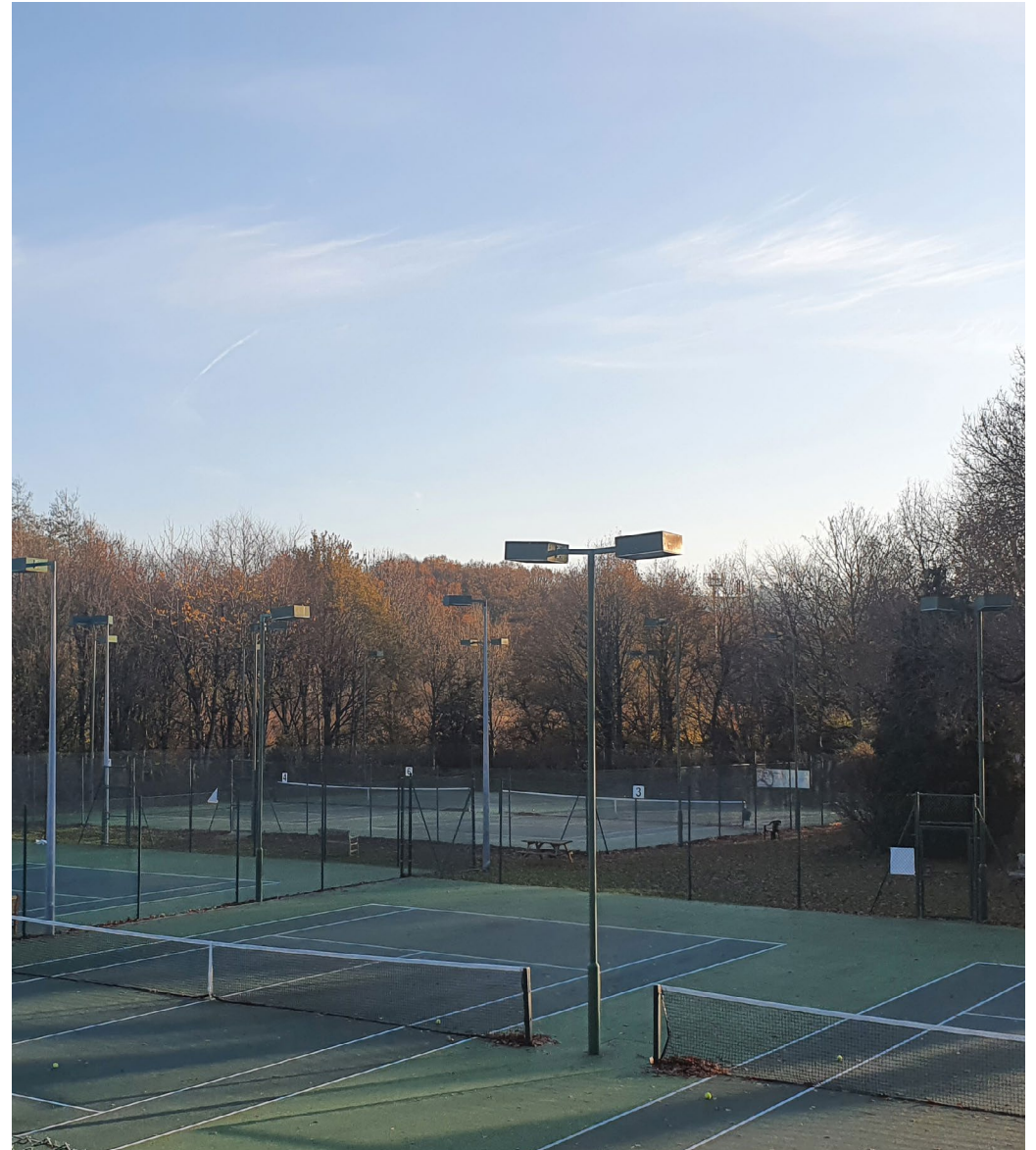
View towards 2no southern courts (Court 7 and 8).
