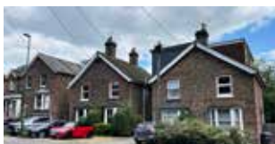
Mill Green Road semi-detached
