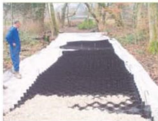
CellWeb during installation.
