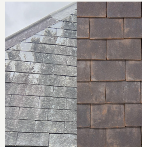
SLATE ROOF TILES / CLAY ROOF TILES (EXISTING)
