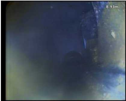
Observation [7]: End Point: INSPECTION CHAMBER -OB
