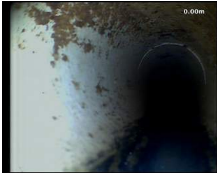
Observation [1]: Start Point: MH1
