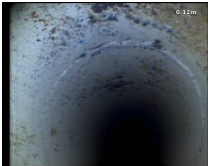
Observation [3]: CRACK
