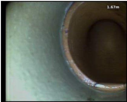
Observation [6]: JDM (BASE OF REST BEND)
