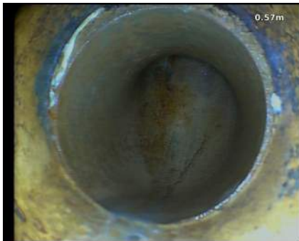
Observation [2]: JDL (BASE OF REST BEND)
