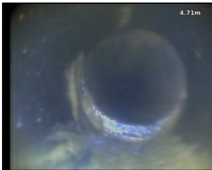
Observation [6]: DROPPED SECTION OF PIPE
