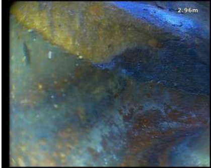
Observation [6]: End Point: MH2
