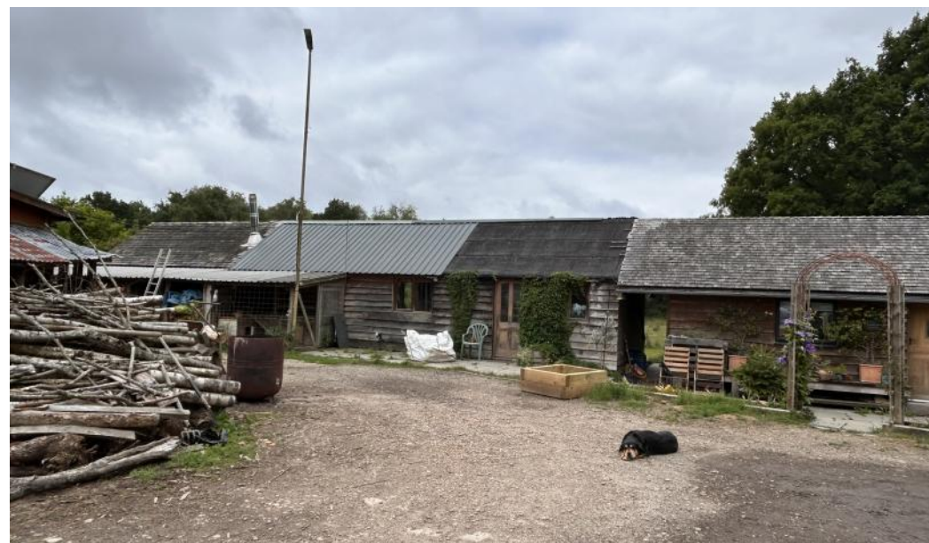
View of front of the old stables comprising Dwelling 1 (RHS) & Dwelling 2 (LHS). Dwelling 1 is to be retained and extended by demolishing Dwelling 2.
