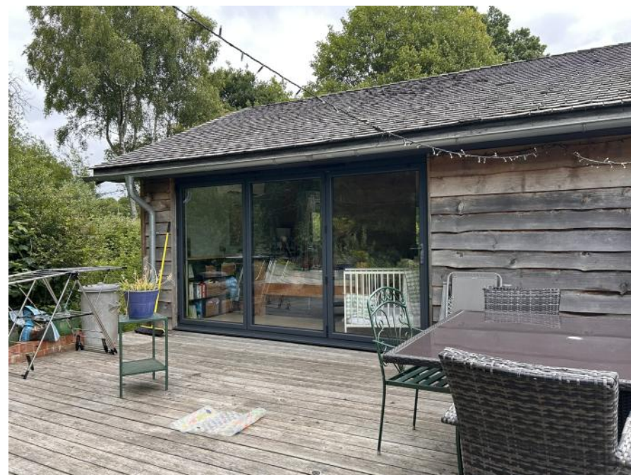
View of rear of Dwelling 1
