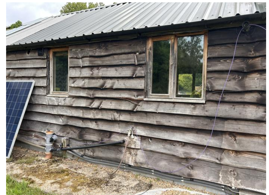
View of rear of Dwelling 2
