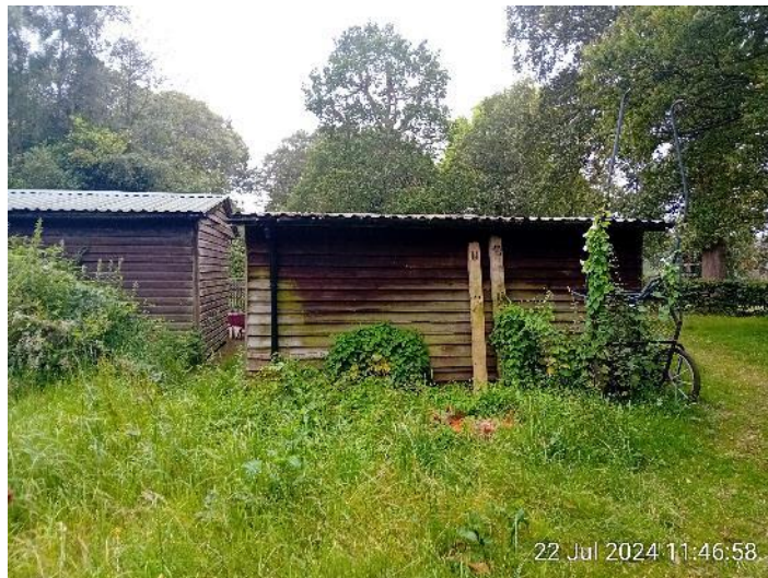
Figure 7: Rear of B2.
