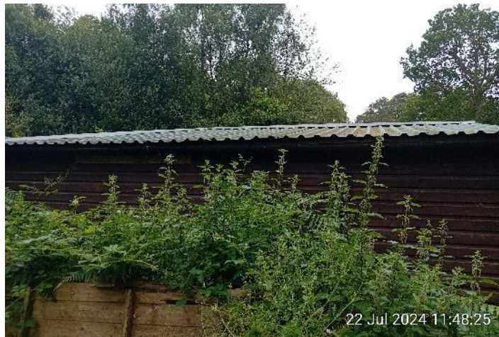
Figure 4: Rear of B1.
