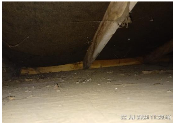
Figure 21: Example of eaves from the interior.
