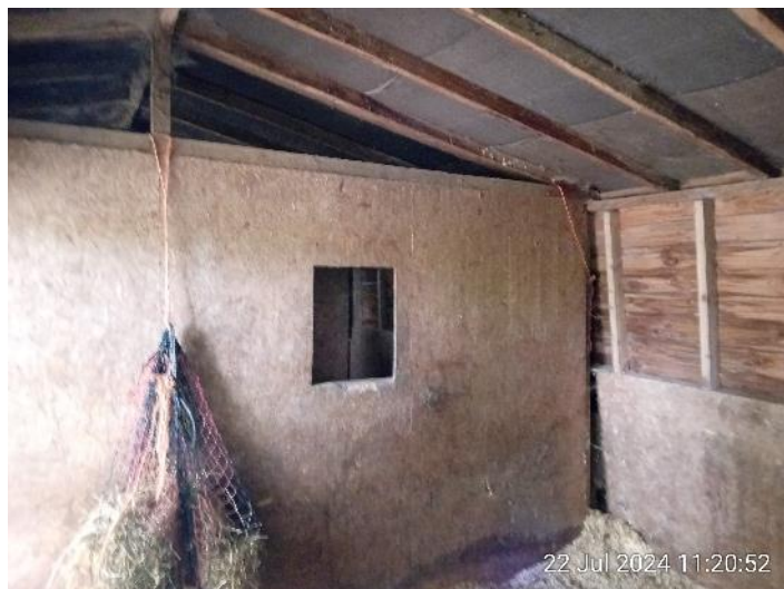
Figure 5: Example of interior of B1.
