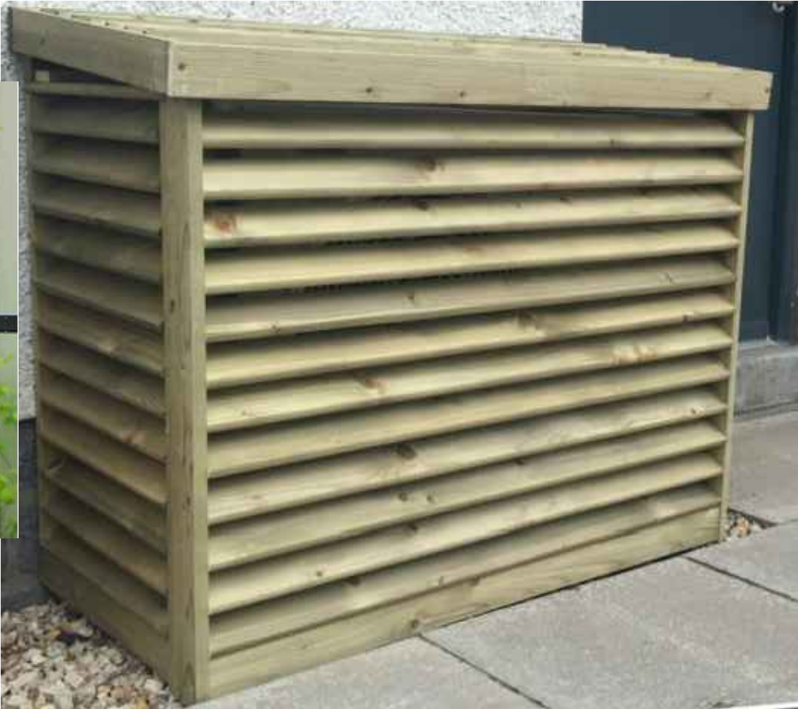
Air Source Heat Pump louvered wooden guard
