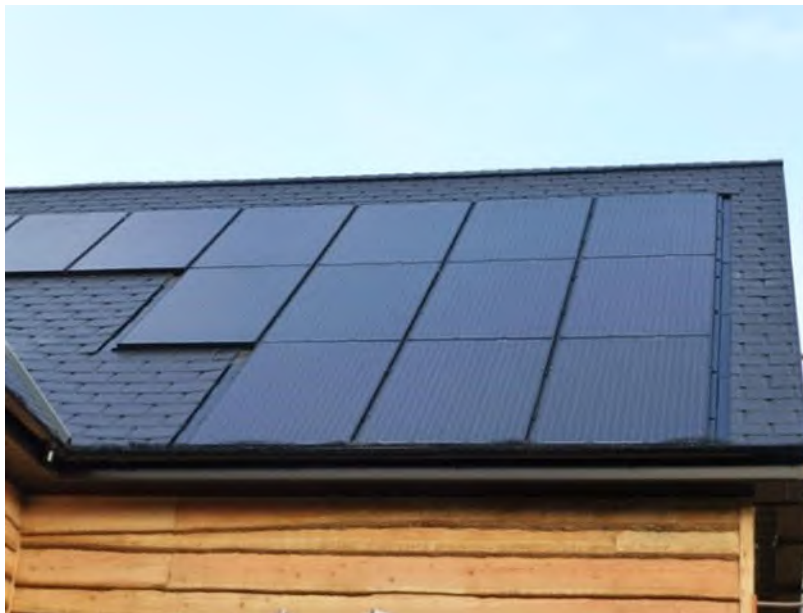
Figure 5.3: In-roof mounting systems
