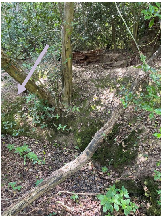
Images 02 & 03 – Showing the 1m+ high embankment at the south-east boundary of the agricultural field. The wet ditch at the base is approx. 1m lower than the field and thus the drain run. The exact location is TBC to suit the path of least resistance through the existing tree line.
