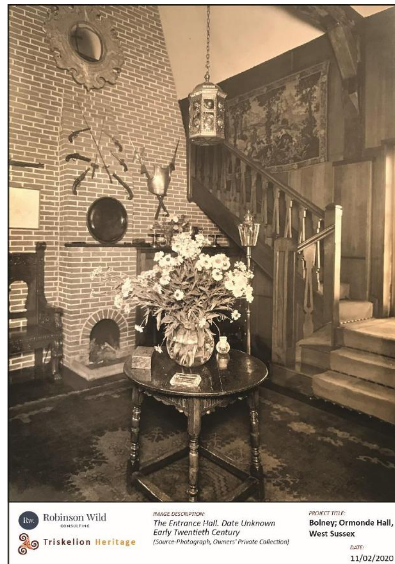
Figure 29 Date Unknown (Early 20 th Century) East Range (the former Old Hall), The Entrance Hall
