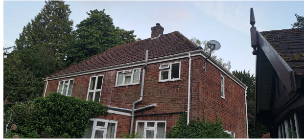
V1 B1-2 surveyor photo
