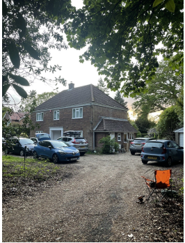
V1 B1-1 surveyor photo
