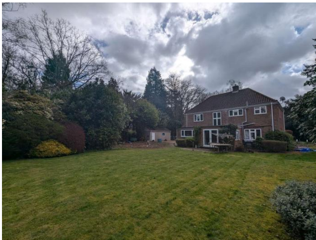
Photo 11: B1 - northern elevation
