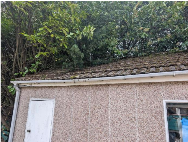
Photo 15: B2 tightly fitted roof tiles.
