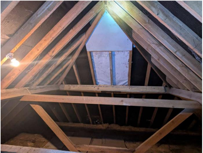
B1 - Internal roof void
