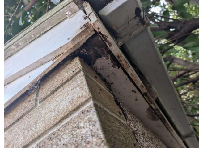
Photo 14: B2 aged but intact soffit boxes
