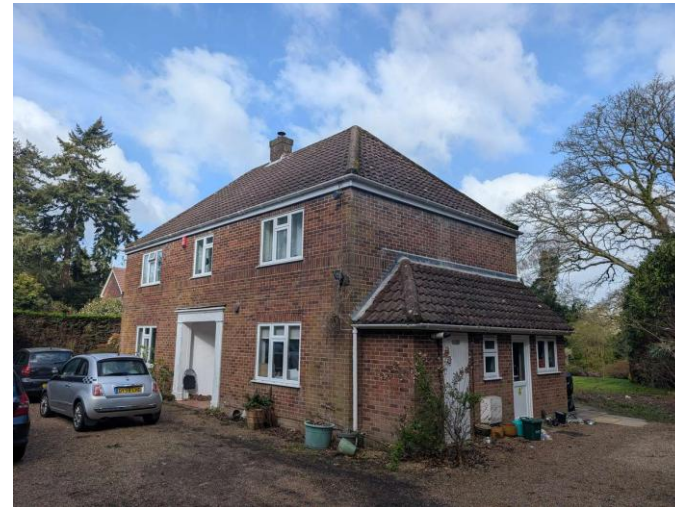
B1 - southeast elevations
