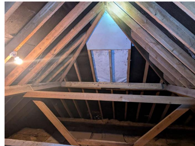
Photo 12: B1 - Internal roof void
