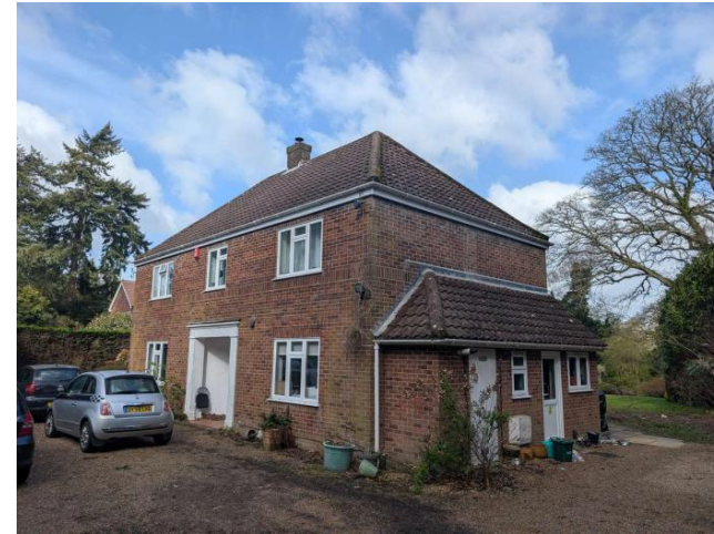
Photo 10: B1 - southeast elevations
