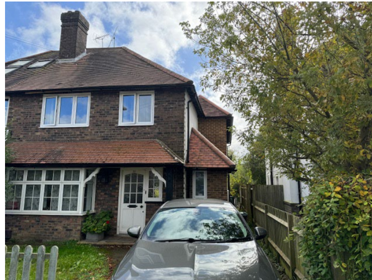
Burgess Hill Dental Practice – existing photos of surrounding side and rear extensions
