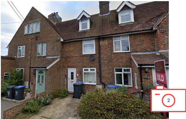
Fig 1.3.02 //Top Road, Neighbourhood dwellings opposite the site
