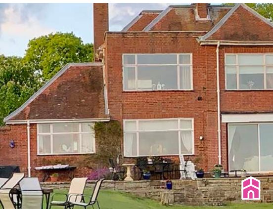
Fig 1.8.03 // Existing South View Building Material Palette
