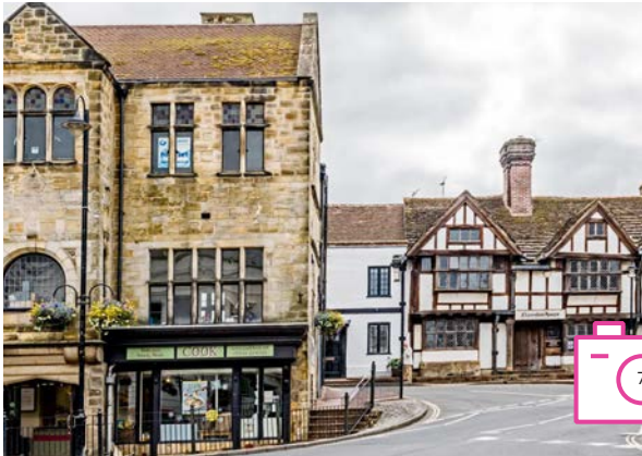
Fig 1.4.01 // East Grinstead Town Centre
