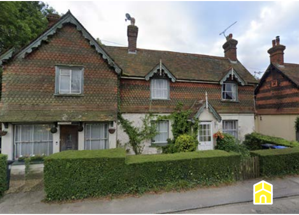
Fig 1.8.10 // 1 & 2 Sharpthorne Villas, Top Road
