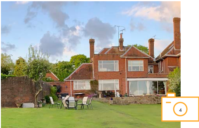
Fig 1.3.04 // The existing dwelling
