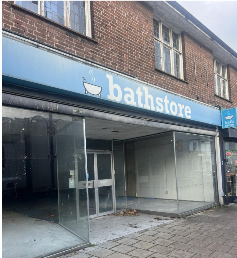
Figure 8: View of the front elevation (top image)
