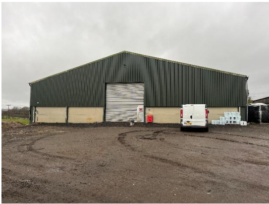
Grainstore front ( east ) elevation
