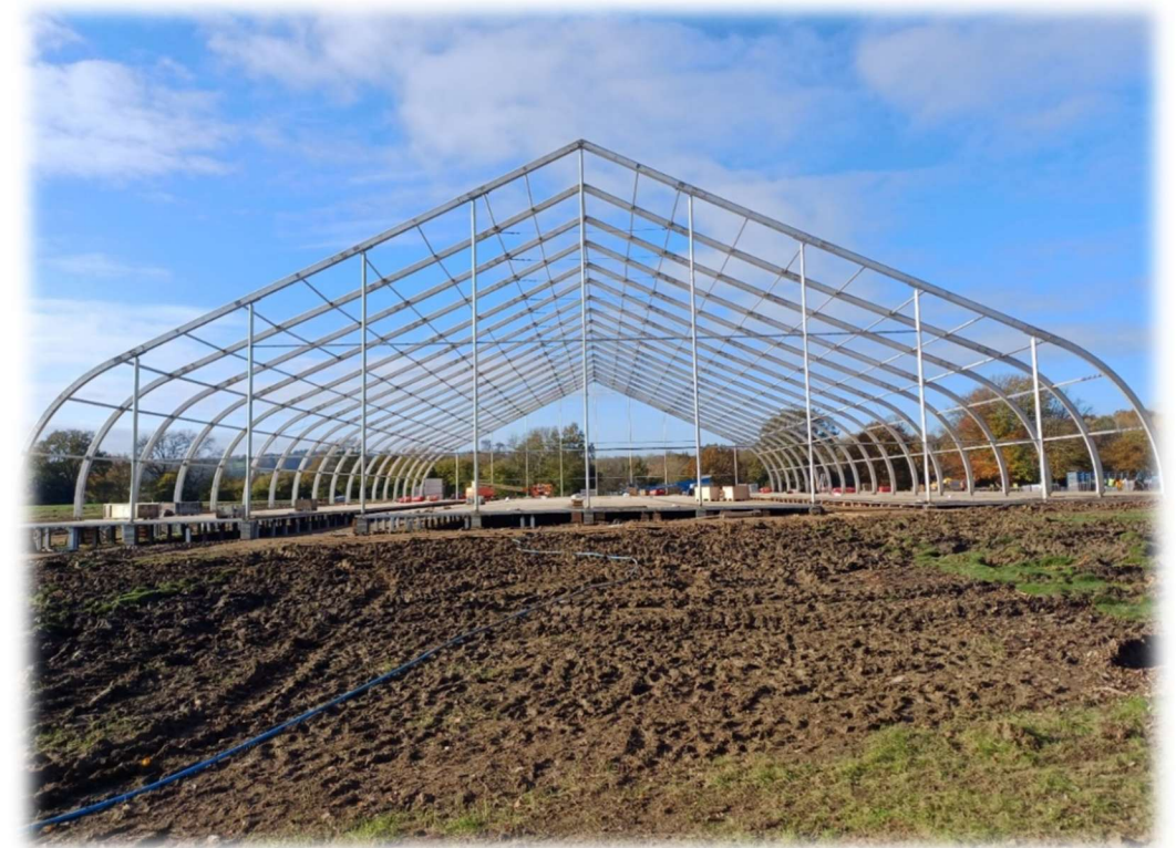
Image 23. Damaged field during event preparation.
