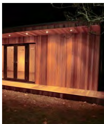
▤ WC block Hobbs Feld / waiting area Juhring Field with integrated lighting
