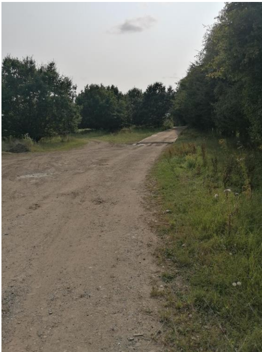
Figure 2.6 Track entrance with start of temporary trackway
