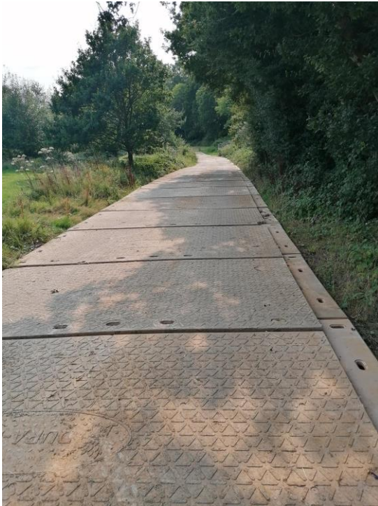
Figure 2.7 Temporary trackway to Hobbs Field
