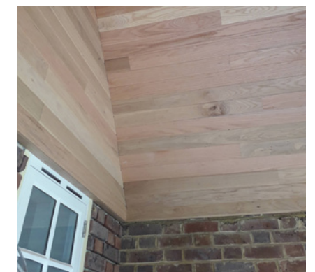
T&G Soffit Cladding
