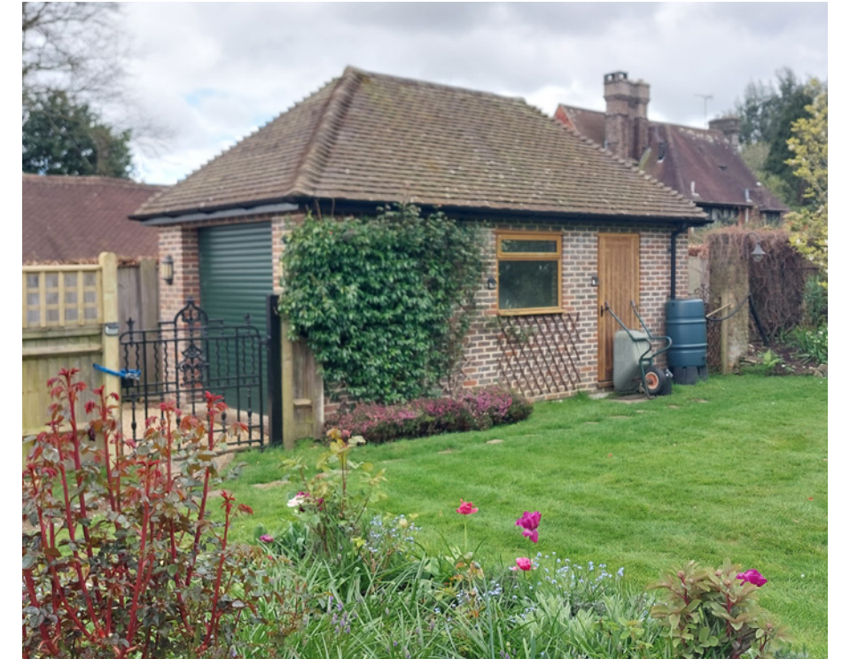
3. Existing Garage as approved under DM/16/2084
