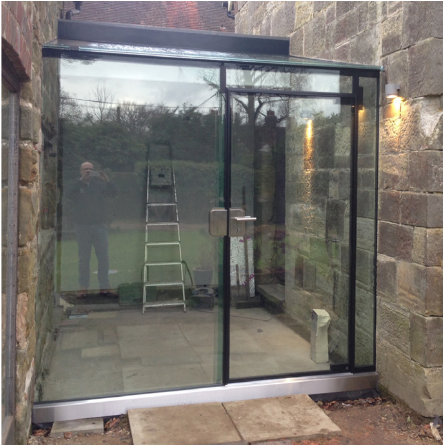
Example of Structural Glazed Link
