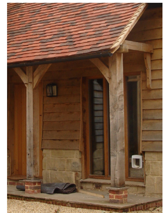
Example of structural oak canopy with open rafter feet and metal gutters
