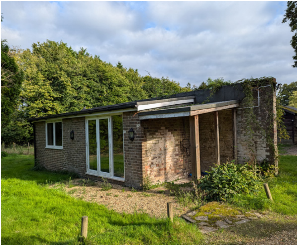
North side of glasshouse wall with lean-to addition
