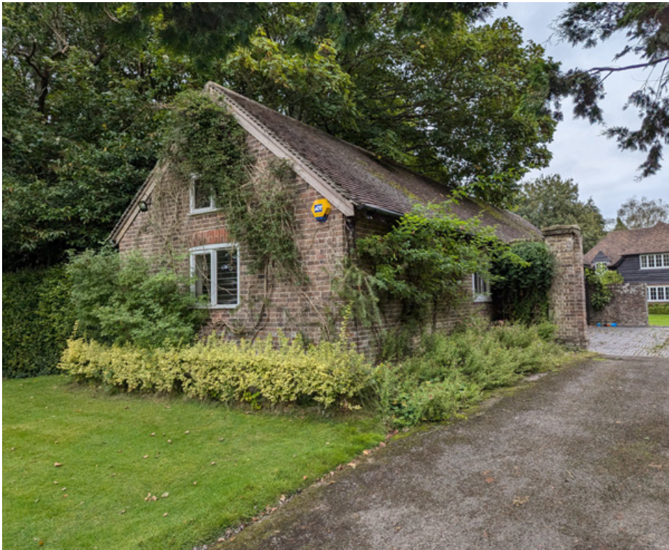
West side of garage to north of courtyard
