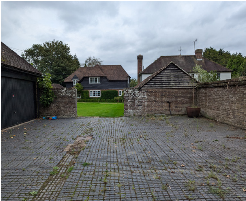
Yard interior looking east
