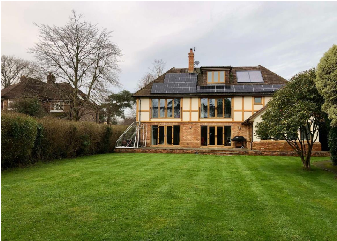
Fig 1: The existing dwelling of Stumble Ridge dates from the early 21 st Century and was built in a tradition mock Tudor style. Vehicular access to the proposed site can be accessed to the side of this dwelling.
