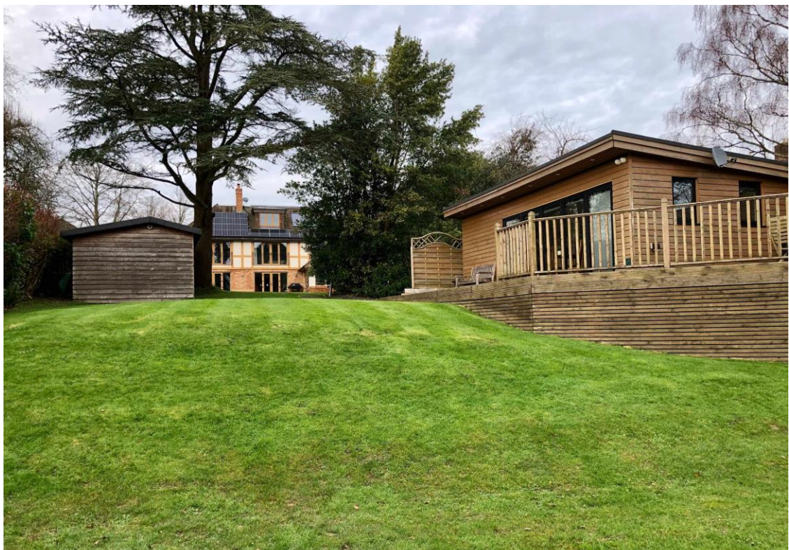
Fig 2: The existing dwelling of Stumble Ridge benefits from a very large rectangular shaped curtilage that extends southwards from Oldlands Avenue. Furthest away, there is a large existing timber clad outbuilding.
