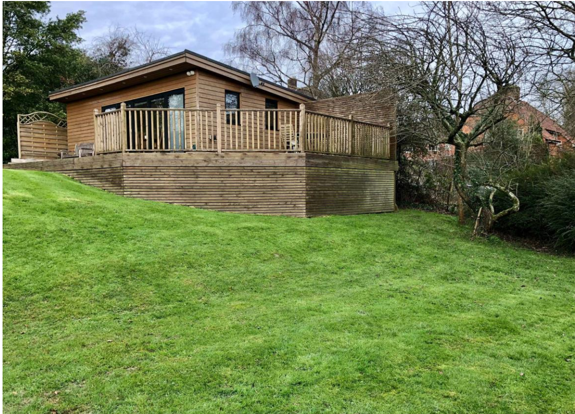
Fig 3: The proposed site sits in a generous existing curtilage space, partly inside of the Balcombe Conservation Area, to the far southern side of the conservation area boundary.
