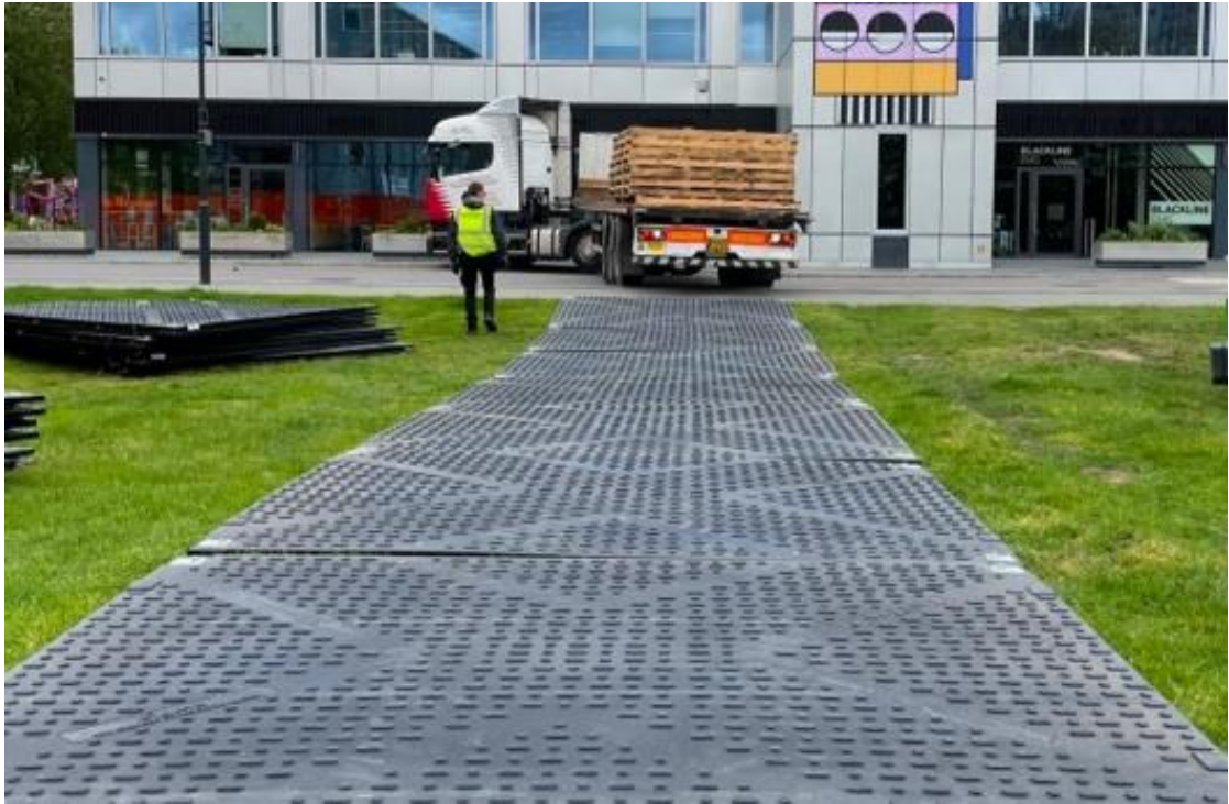
Figure 6 – Example of temporary trackway panels used to create a temporary trackway to the site.
