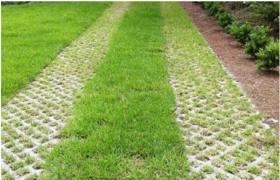
Figure 7 – Example of a ribbon strip reinforced surface solution for existing access post development if required.
