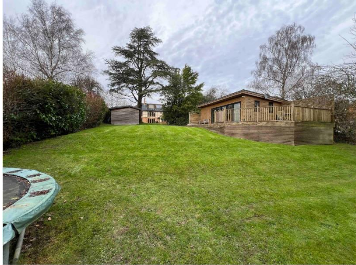
Figure 4 - View of existing outbuildings from the south
