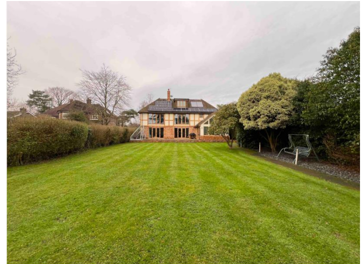
Figure 7 - South elevation of Stumble Ridge (taken from north of outbuildings)
