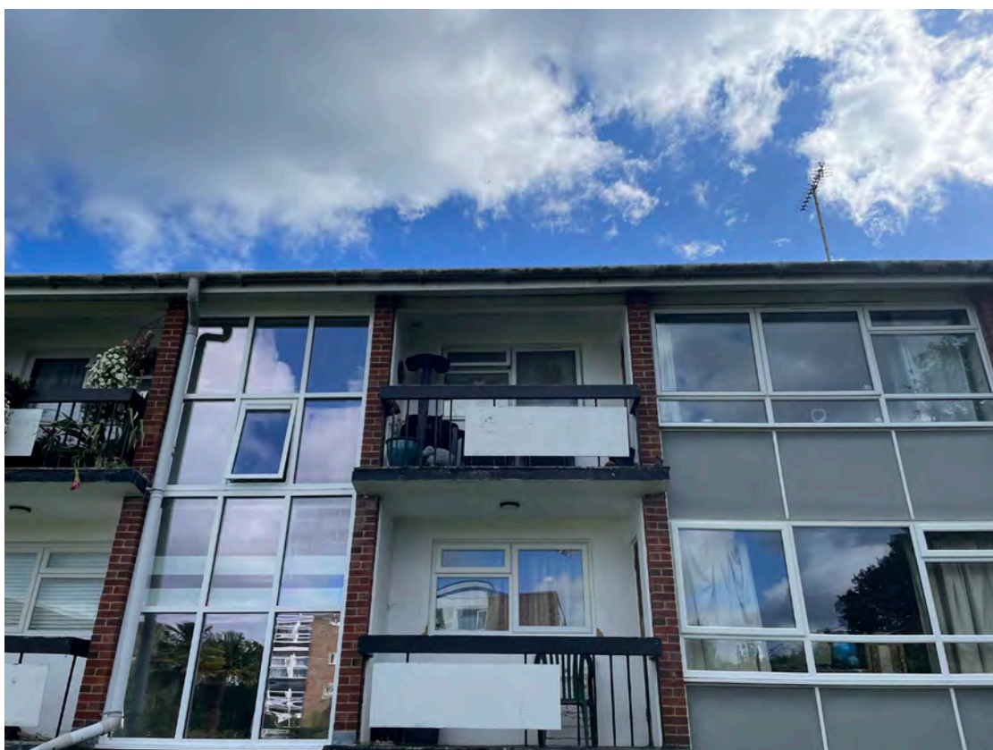
30 - Closer view of No.12 Byron Court Balcony (top floor)
