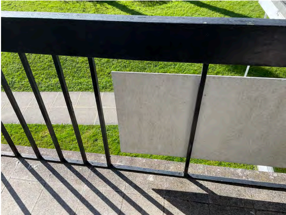
7 - No. 4 Chaucer Court Balcony front section with infill panel
