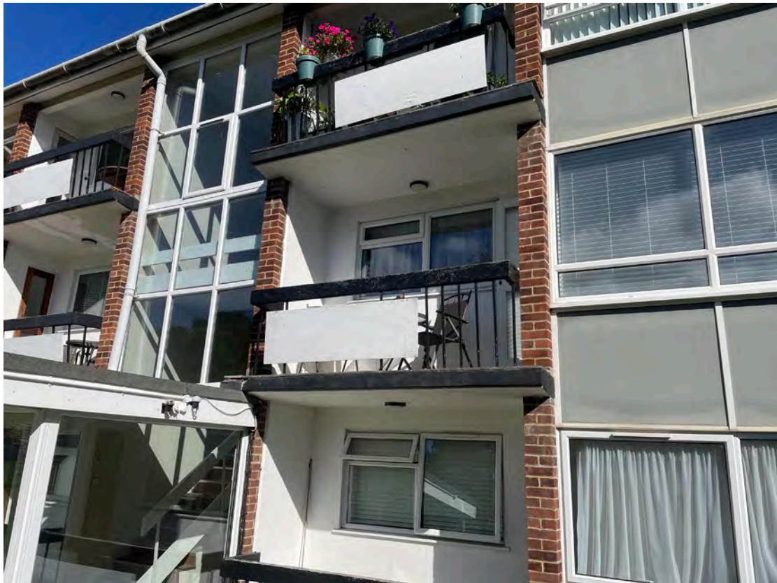
15 - Closer view of No.10 Chaucer Court Balcony
