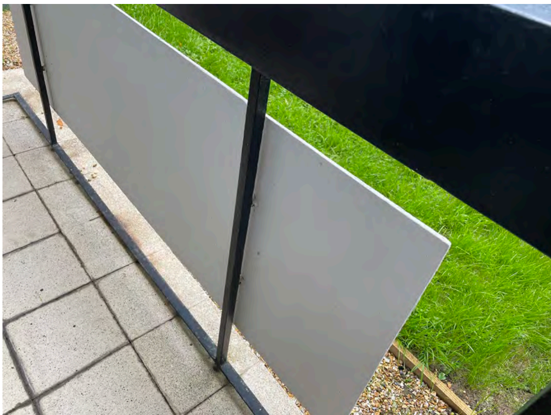
26 – No. 8 Byron Court Balcony front infill panel
