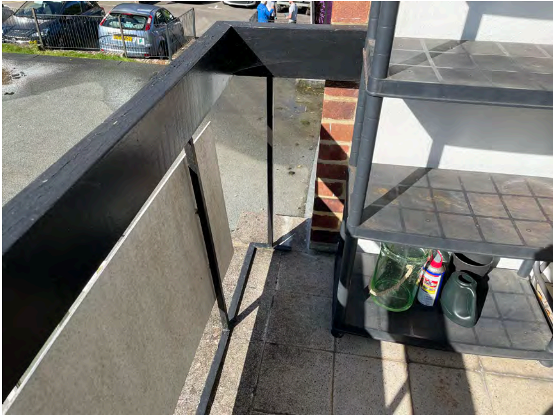
9 - No. 4 Chaucer Court Balcony west side return
