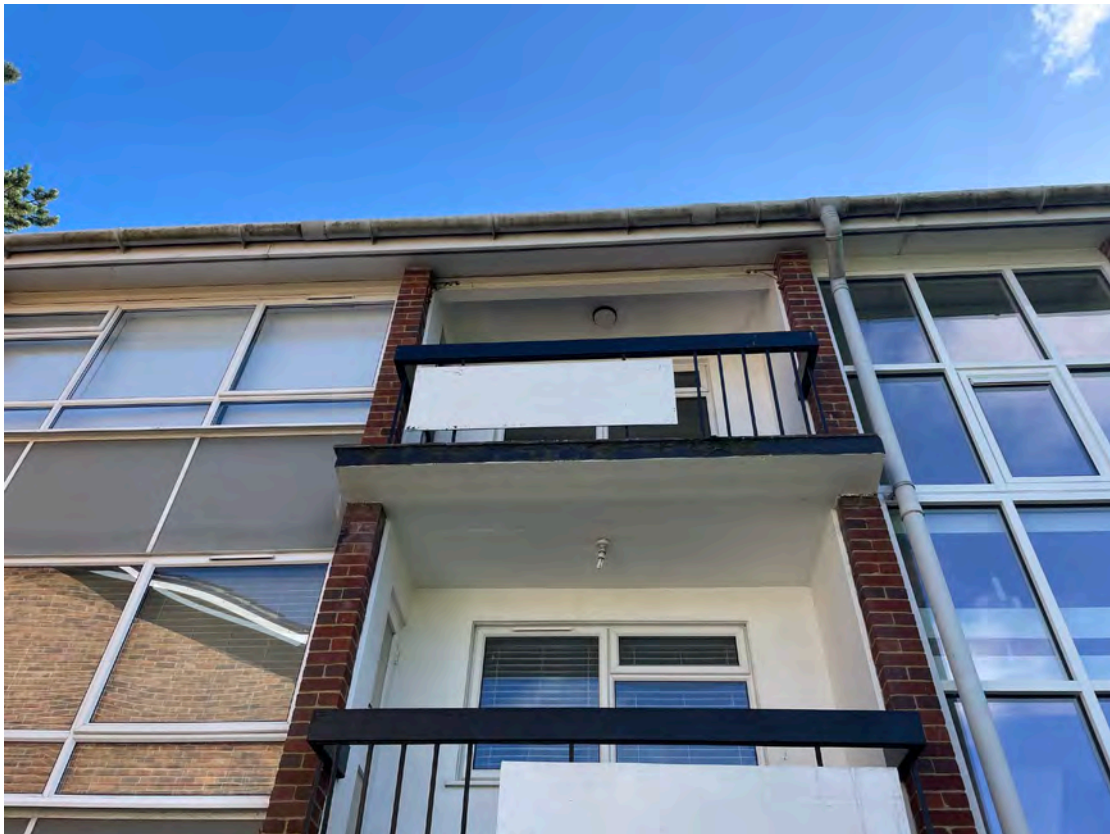
20 - Closer view of No.5 Byron Court Balcony (top floor)
