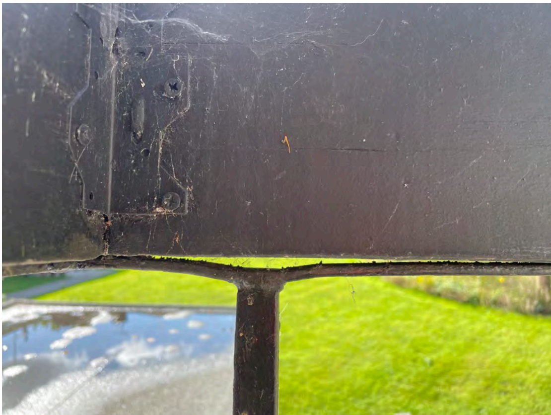
14 - No. 9 Chaucer Court Balcony east side extra post top welded connection
