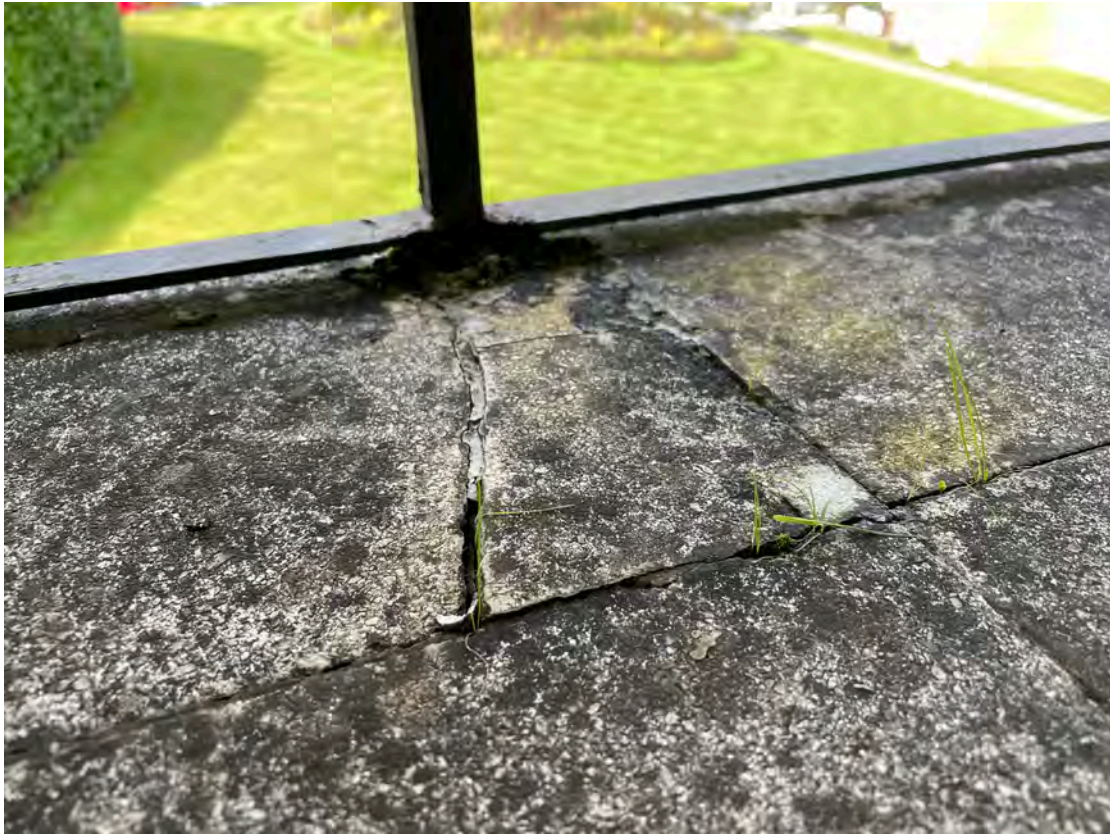
33 – No. 12 Byron Court Balcony front bottom rail corrosion and cracked paving slab
