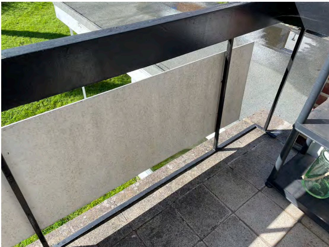
8 - No. 4 Chaucer Court Balcony west side
