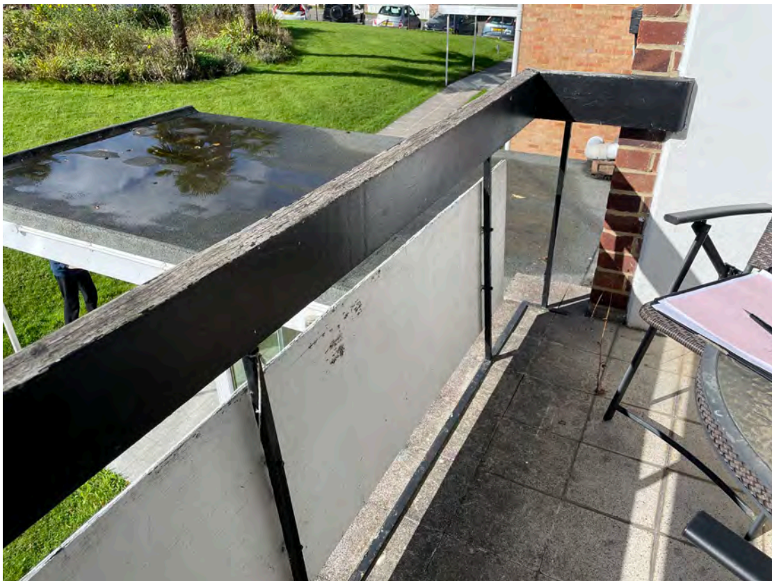
18 – No. 10 Chaucer Court Balcony west side
