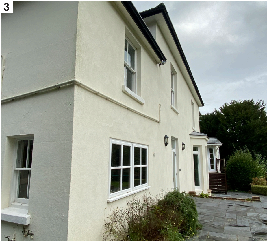
Corner of South and West Elevations, Facing East
