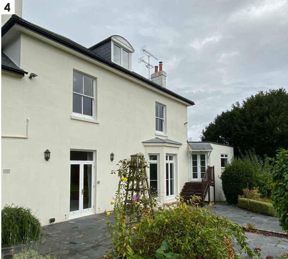
South Elevation, View to North-East
