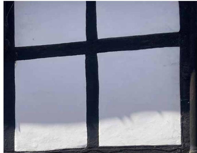
Black painted timber frame with white painted plaster infill
