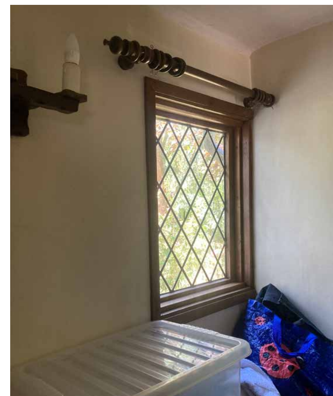
Photograph of existing entrance porch window (interior)
