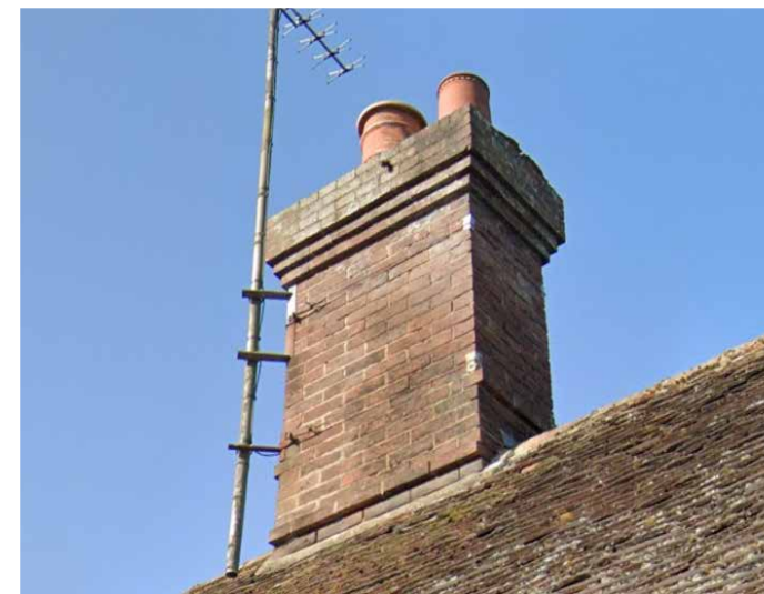
Red brick chimney
