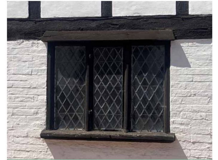
Timber framed window with diamond pattern leaded glazing
