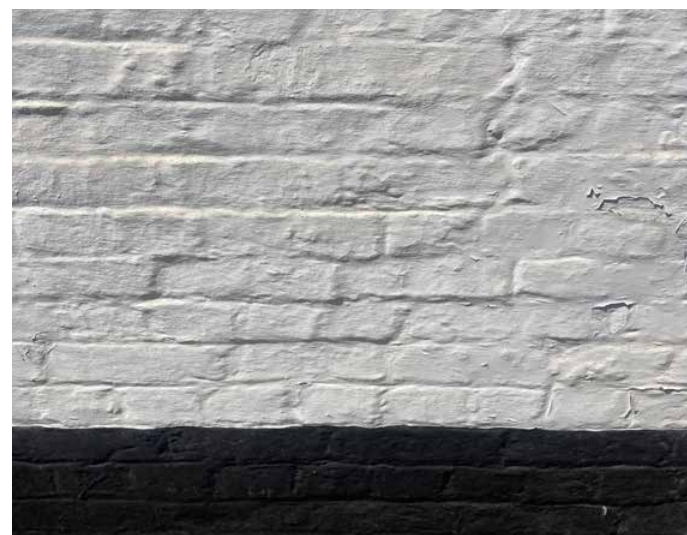
White painted brick walls
