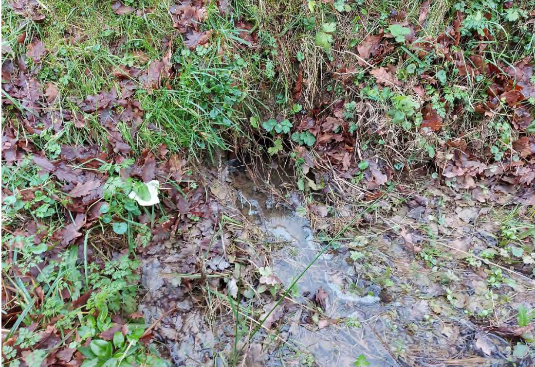
Photo 3: Culvert outlet from receiving ditch entering ditch on opposite side of access road, viewed from the east
