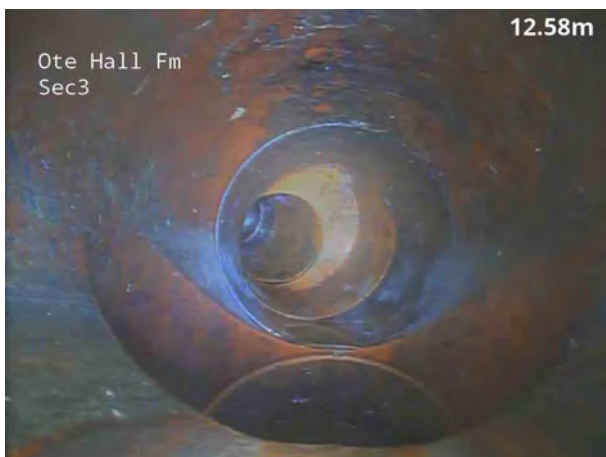
5, 00:00:45, 12.60 m Line deviates down, At tumbler
