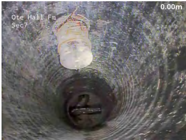
1, 00:00:00, 0.00 m Start node, manhole, reference: FW2
