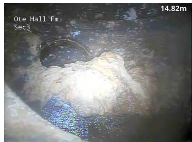
6, 00:01:09, 14.80 m Finish node, manhole, reference: FW2
