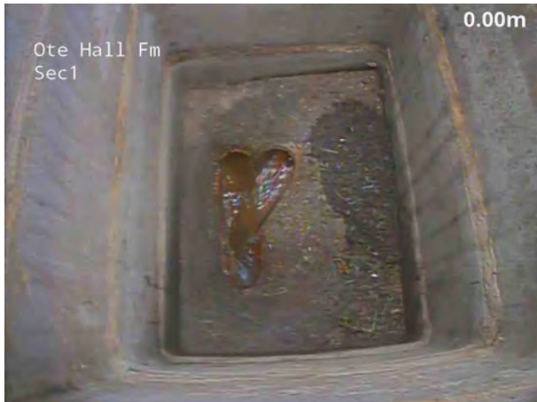
1, 00:00:00, 0.00 m Start node, manhole, reference: FW1
