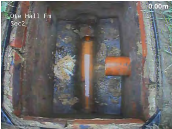
1, 00:00:00, 0.00 m Start node, manhole, reference: FW4
