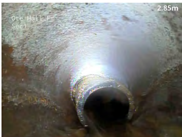
3, 00:00:46, 2.90 m Pipe size changes, new size(s), 50mm high
