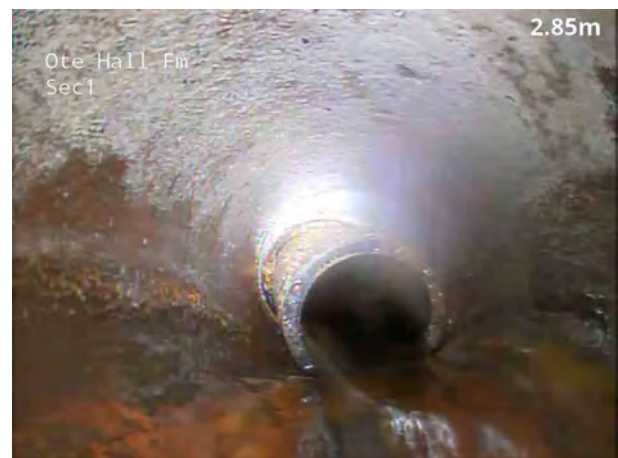
4, 00:01:08, 2.90 m Finish node, manhole, reference: Pump, To pump outlet
