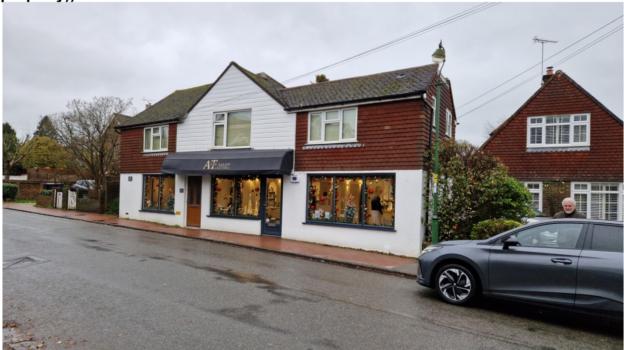
Figure 1: External view (from south – note UPVC windows to neighbouring property))
