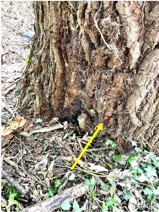
T206 Poplar spp. Looking West towards measurements drill location No.7
